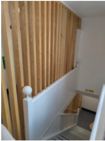
Image of the existing open timber slat screen to Stair 2 on the first floor.
