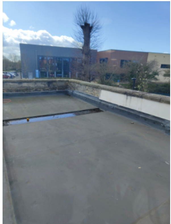
Image of the existing flat roof to the plant room where the new AC unit is proposed.
