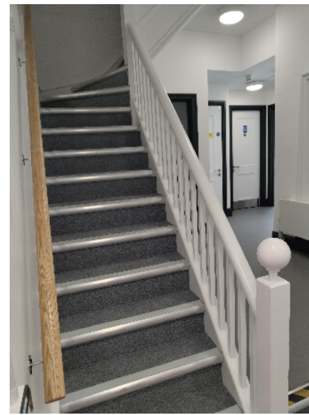
Figure 1: Existing photo of Stair 3
