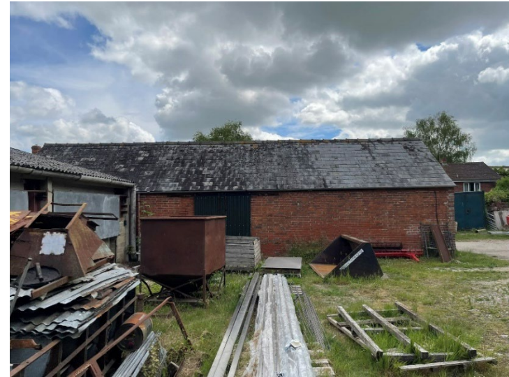
Plate 36: Western elevation of Barn 6.
