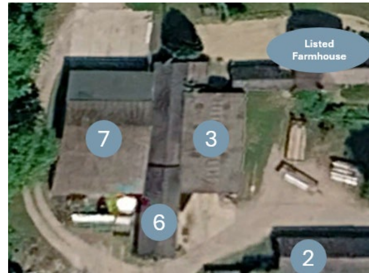
Plate 23: Site layout extract showing location of Barn 3.
