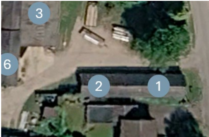
Plate 18: Site layout extract showing location of Barn 2.
