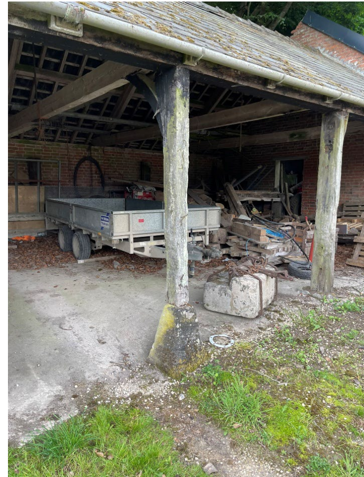
Plate 27: Barn 4, bracketed post supports.
