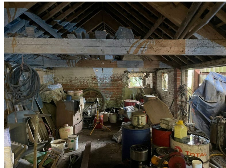
Plate 38: Barn 6's central internal section.
