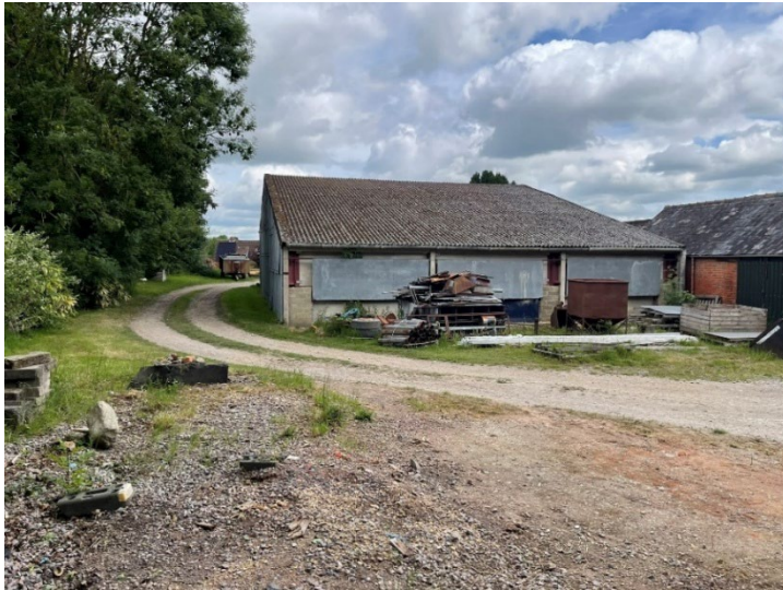
Plate 41: Barn 7's southern elevation.
