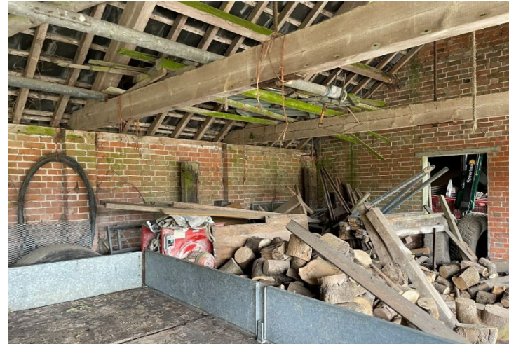
Plate 28: View towards the southern western internal elevation of the barn.
