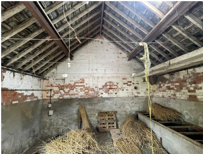
Plate 17: the eastern interior wall of Barn 1.
