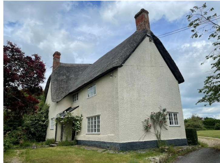
Plate 43: Old Manor Farm Farmhouse's southern and eastern elevations as seen from the front entrance.
