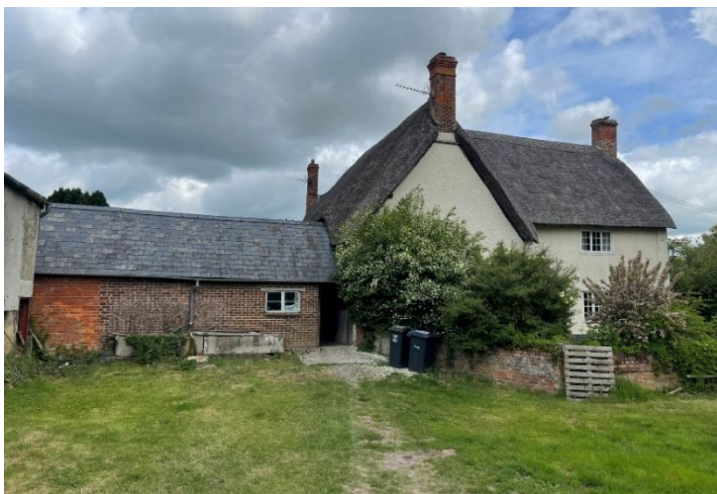
Plate 45: View of the farmhouse's southern elevations from the courtyard of the farm.
