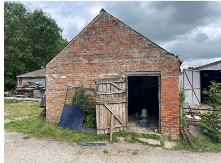
Plate 34: Barn 6's Southern Elevation.
