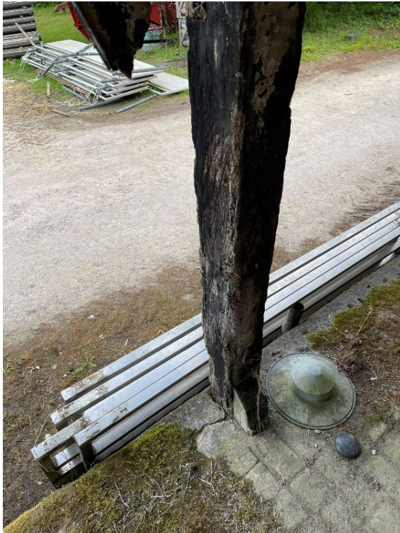
Plate 20: Barn 2, detail of post.
