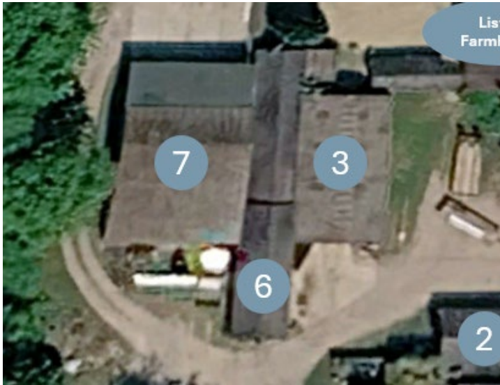
Plate 33: Site layout extract showing location of Barn 6.
