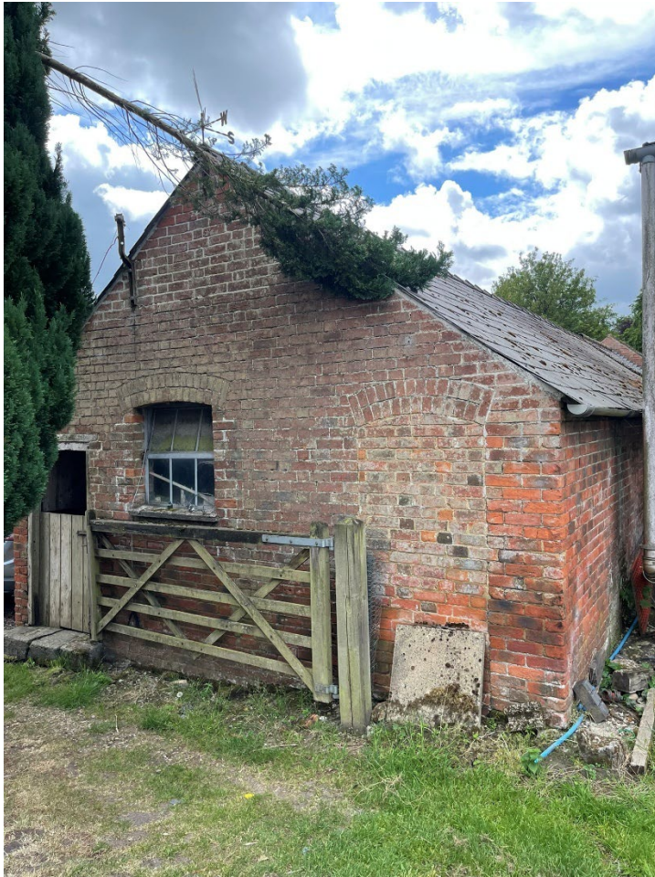
Plate 39: Barn 6's northern elevation, showing segmental arches and brickwork.
