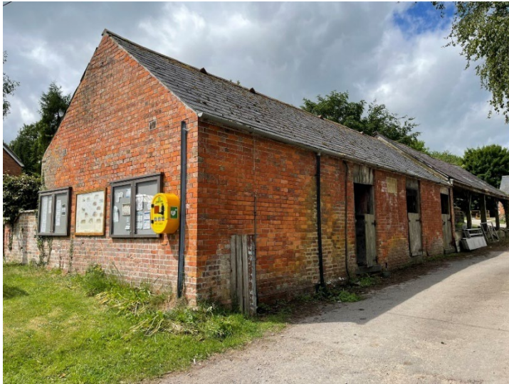
Plate 14: Barn 1, eastern and northern elevations as seen from the High Street.
