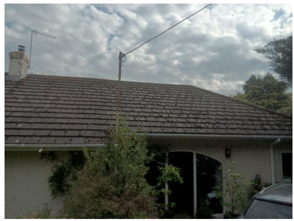
Plate 2. Front elevation of B1.
