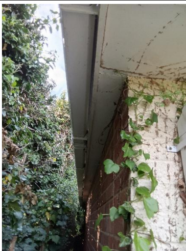
Plate 5. Soffit boxes in good condition around whole of B1.
