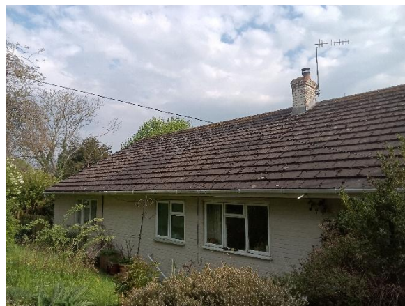
Plate 1. Rear elevation of B1.
