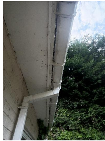
Plate 4. Soffit boxes in good condition around whole of B1.
