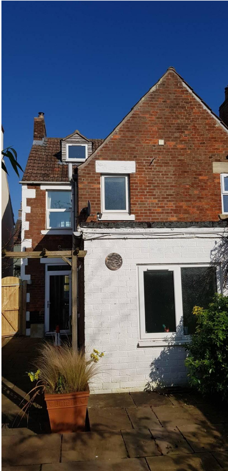
Existing Rear Southwest Elevation.
