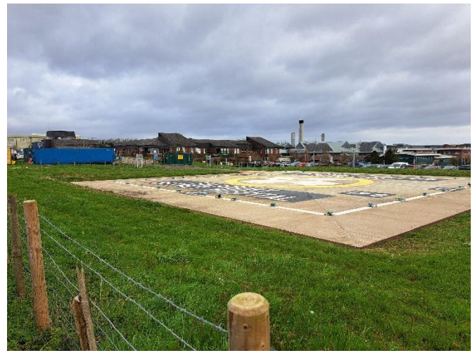
Photograph 12. Helipad and grassland in south of site. March 2026.
