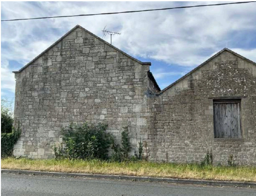
Plate 1. Rear elevation (facing north and adjacent to Bradford Road)
