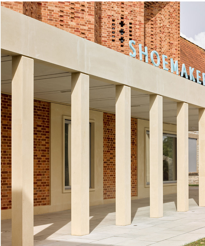
Wet Cast Stone - New Extensions
