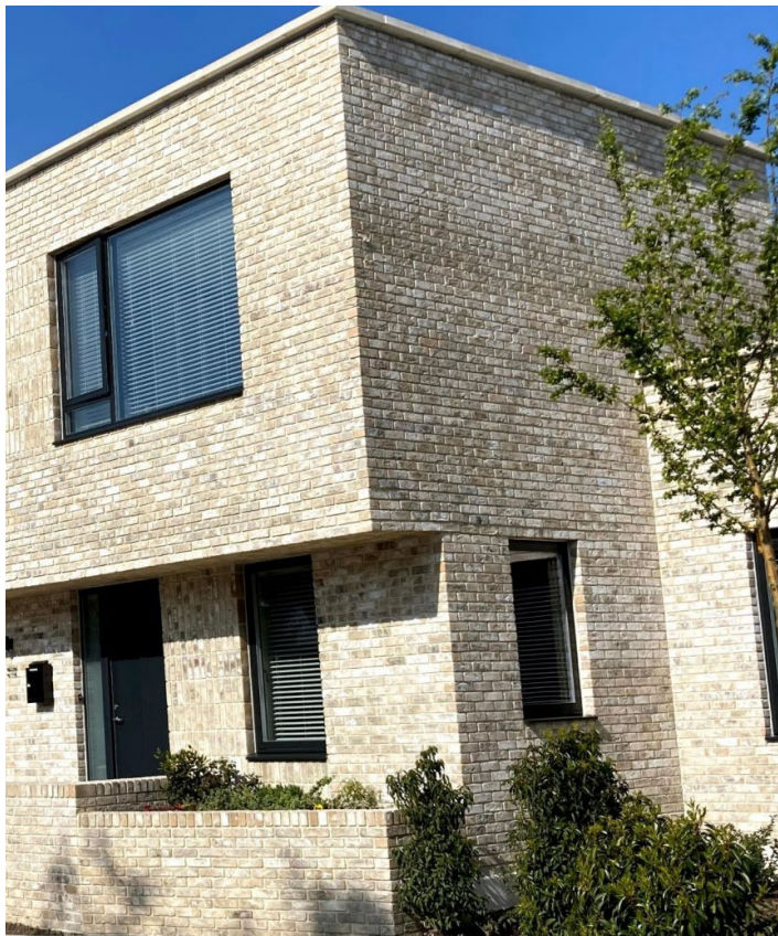
Facing Brickwork and Pointing - New Extensions
