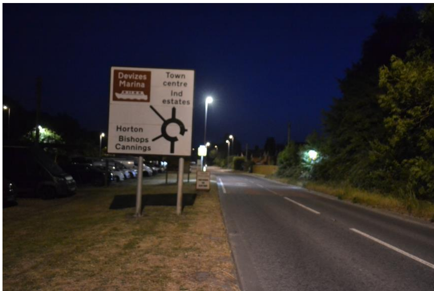
Photograph 15: View along the A361/London Road towards the A361/Horton Road roundabout, showing the existing highway lighting columns and direction signage. Taken at 22:37 on 16 July 2026 (1/4 sec, f/3.5, ISO 3200).
