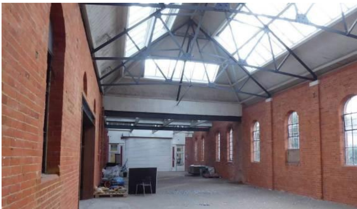
Fig 3.4: Area 4 looking in to area 3
