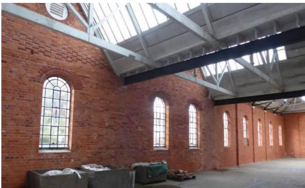
Fig 3.3: Area 3, looking in to area 4
