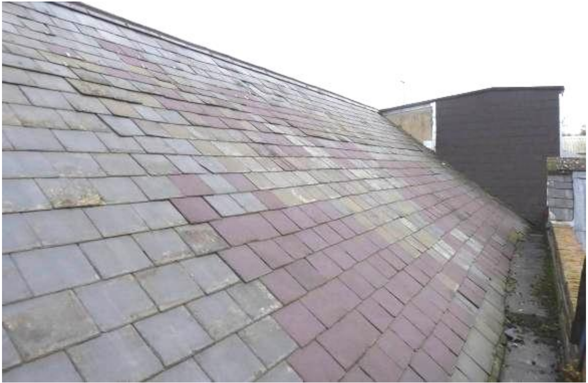
Fig 4.5: Area 5 roof, south side
