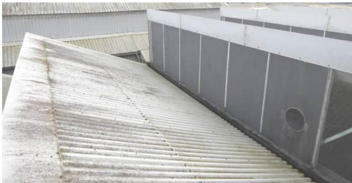
Fig 3.1.13: Area 1 north light roofs
