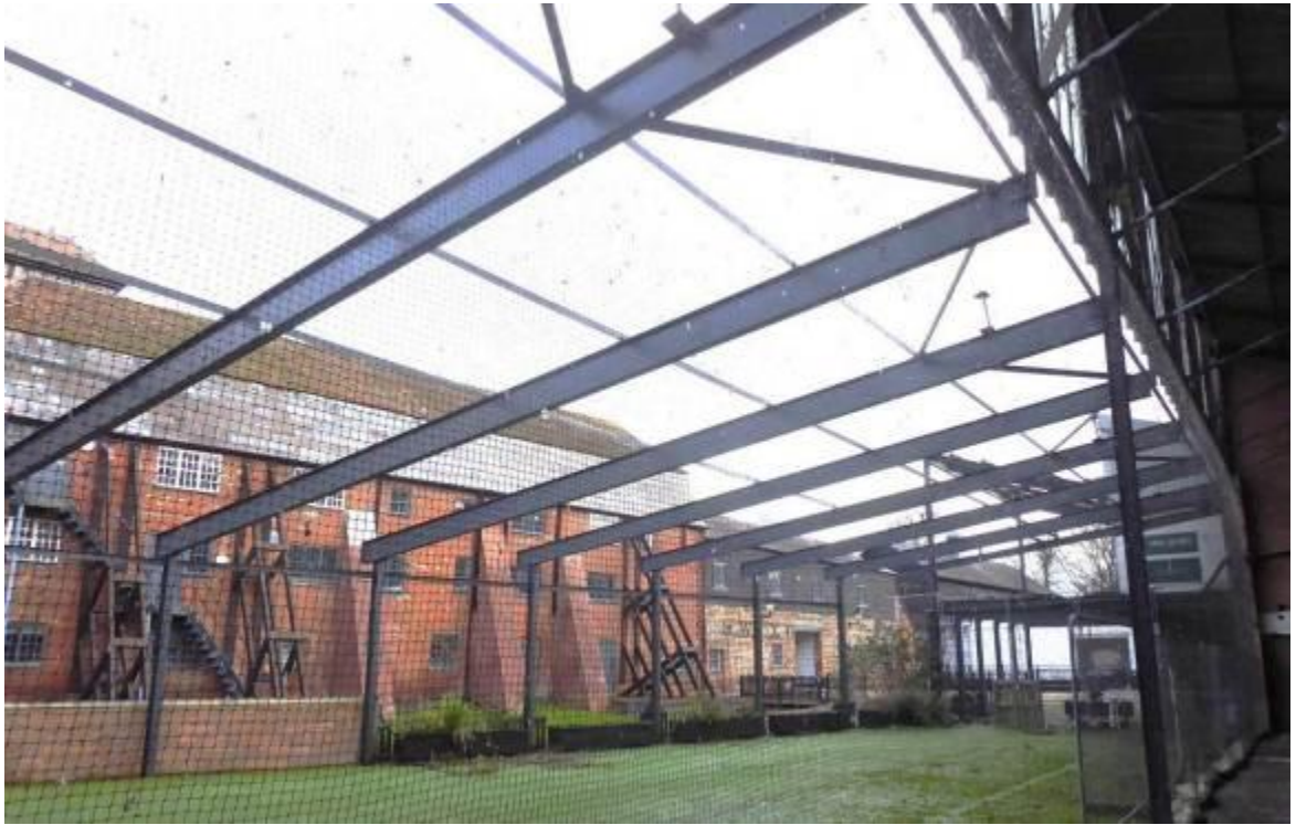
Fig 3.8.2: Area 8 from area 7, looking northeast
