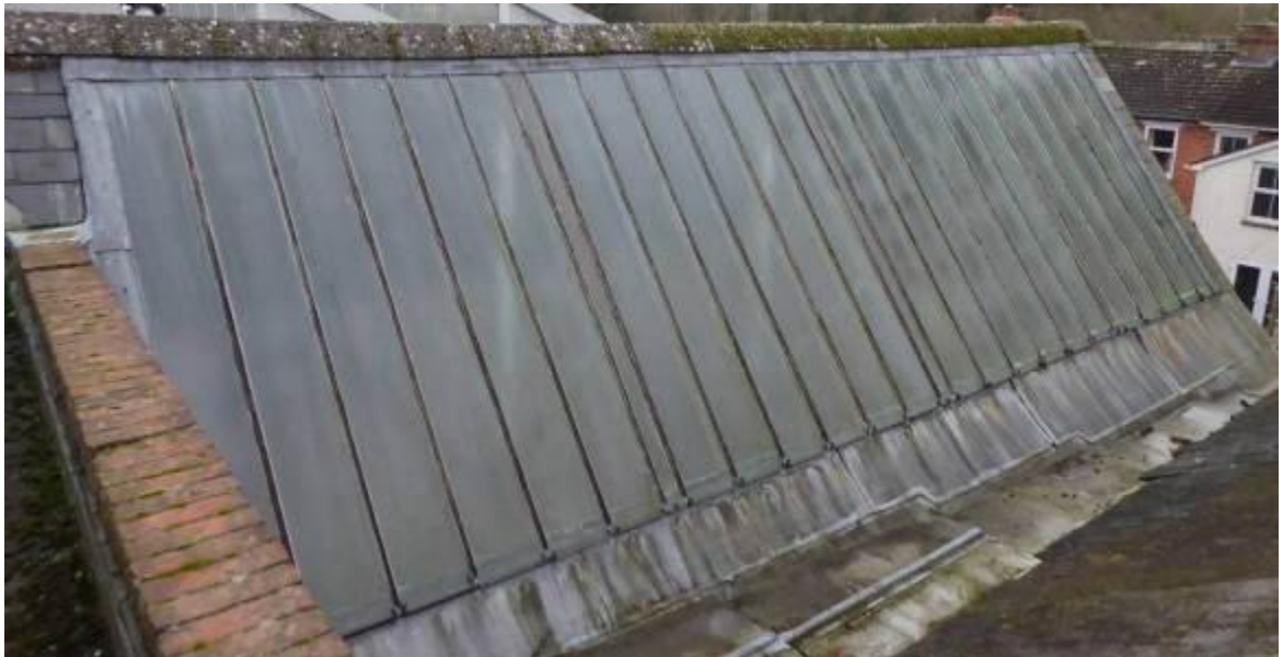
Fig 3.3.7: West light to roof over area 3
