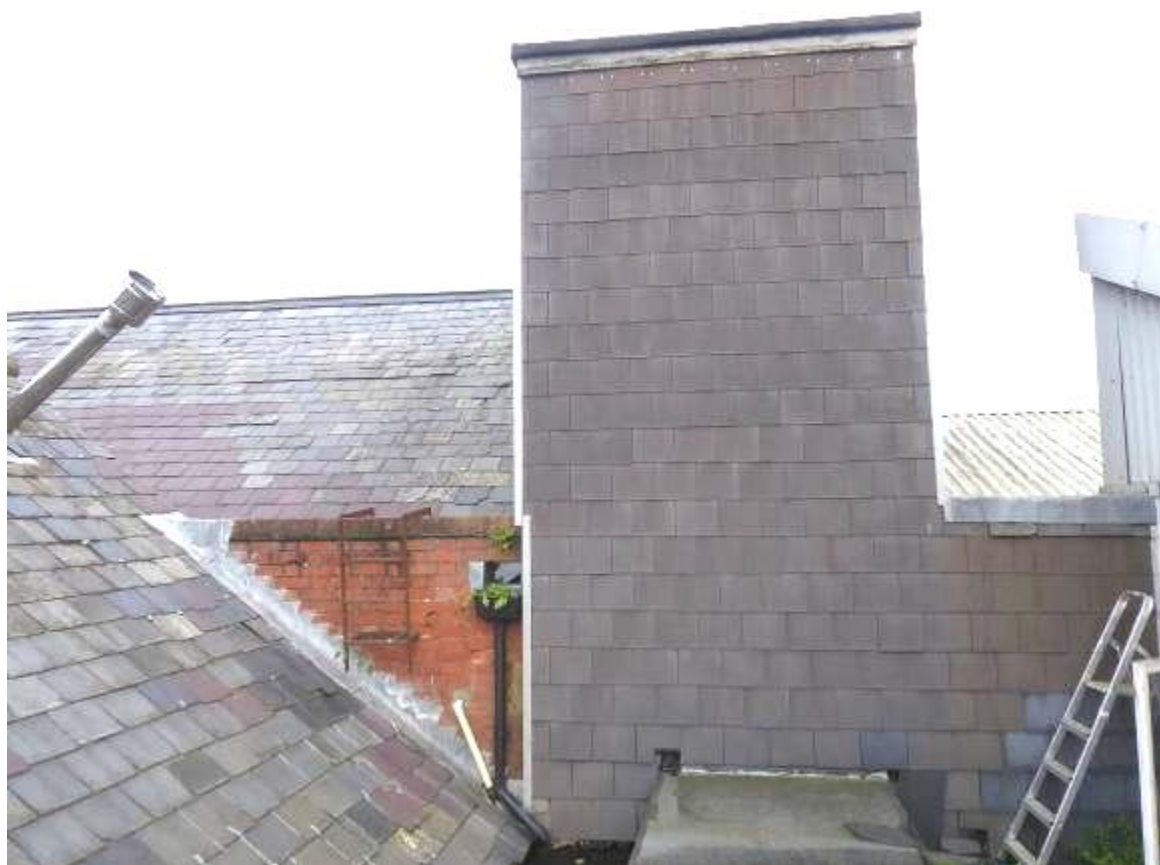
Fig 3.1.12: Lift shaft and south side of area 5 roof
