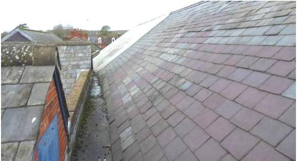
Fig 3.3.7: Valley gutter between roofs to areas 3 and 5
