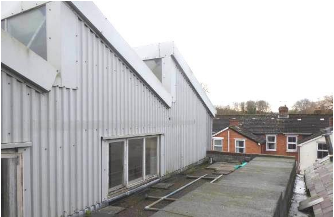
Fig 3.1.12 West side of area 1 roof
