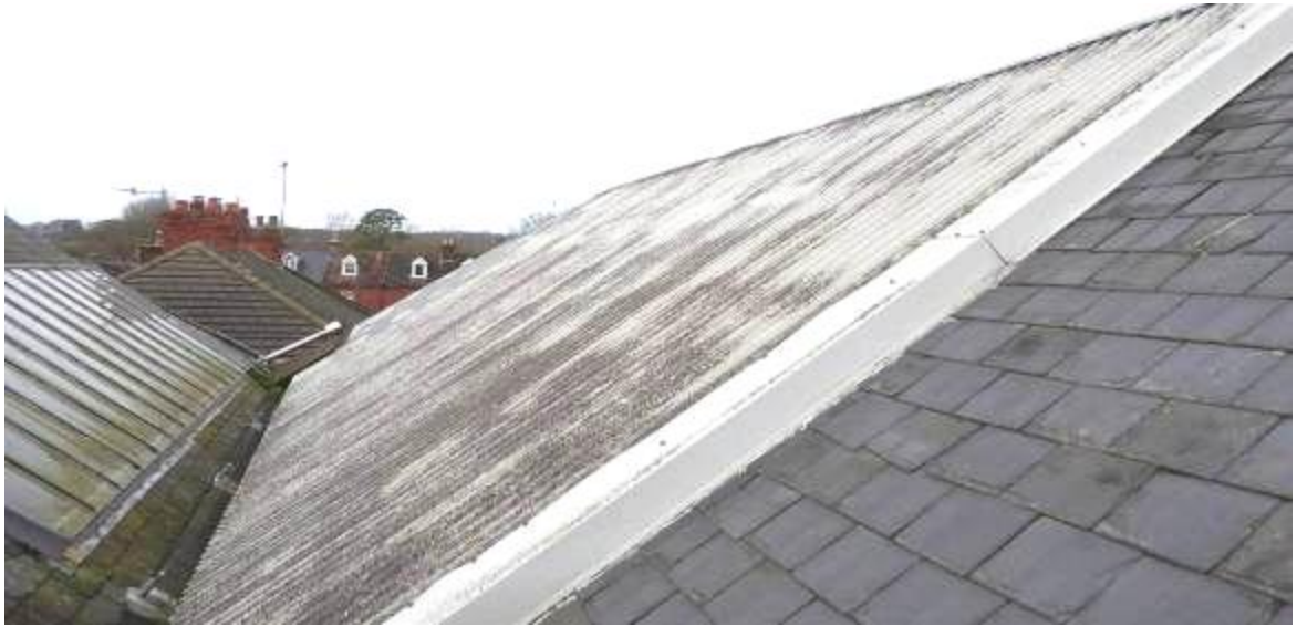
Fig 3.6.5: Area 6 south roof slope
