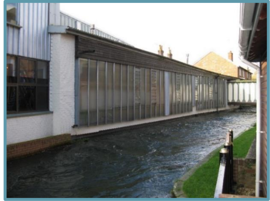
Photo 2 - Façade Units 5B, 5C & 5D (looking west).
