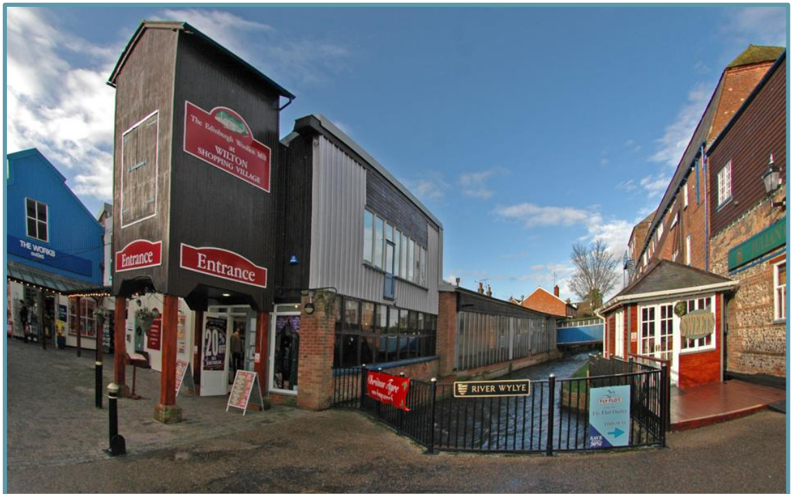
Figure 5 Former façade viewed from northeast prior to removal of cladding, shows tower, which has also been removed, and entrance set back
