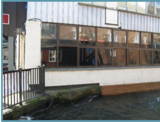
Photo 1 - Façade Unit 5A (Looking west).
