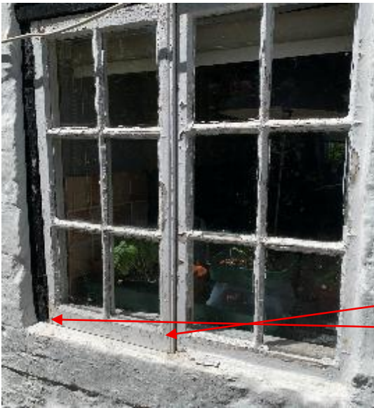
View of exterior kitchen window W2
