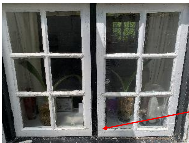
Rear Sitting Room Window (exterior) W1
