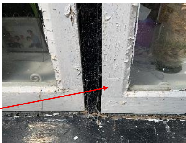
Example of previous repair work
