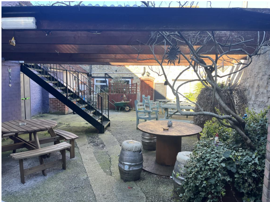
Fig.4 Existing Timber Pergola Roof
