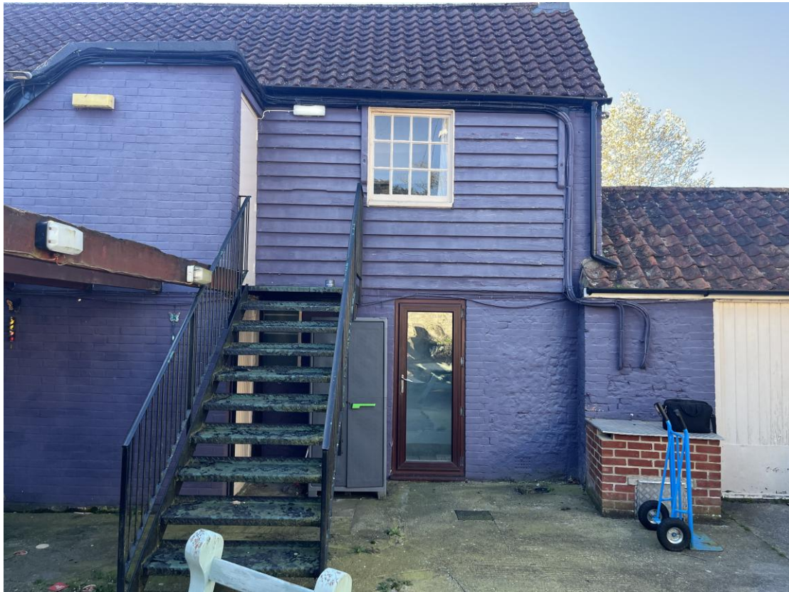
Fig.3 Existing Function Room Staircase and Fire Escape
