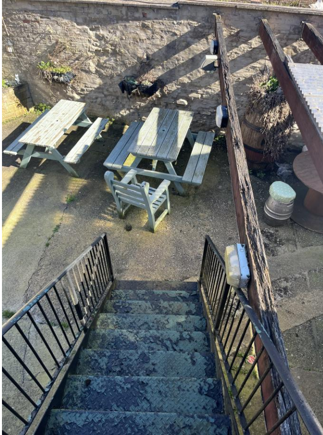
Fig.1 Existing Fire Escape
