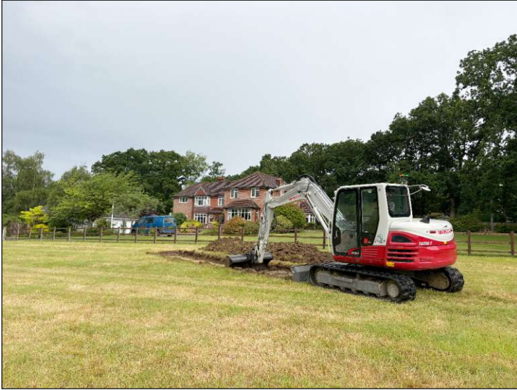
Plate 1: Working view during excavation of Trench 1. Looking northwest towards The Uplands
