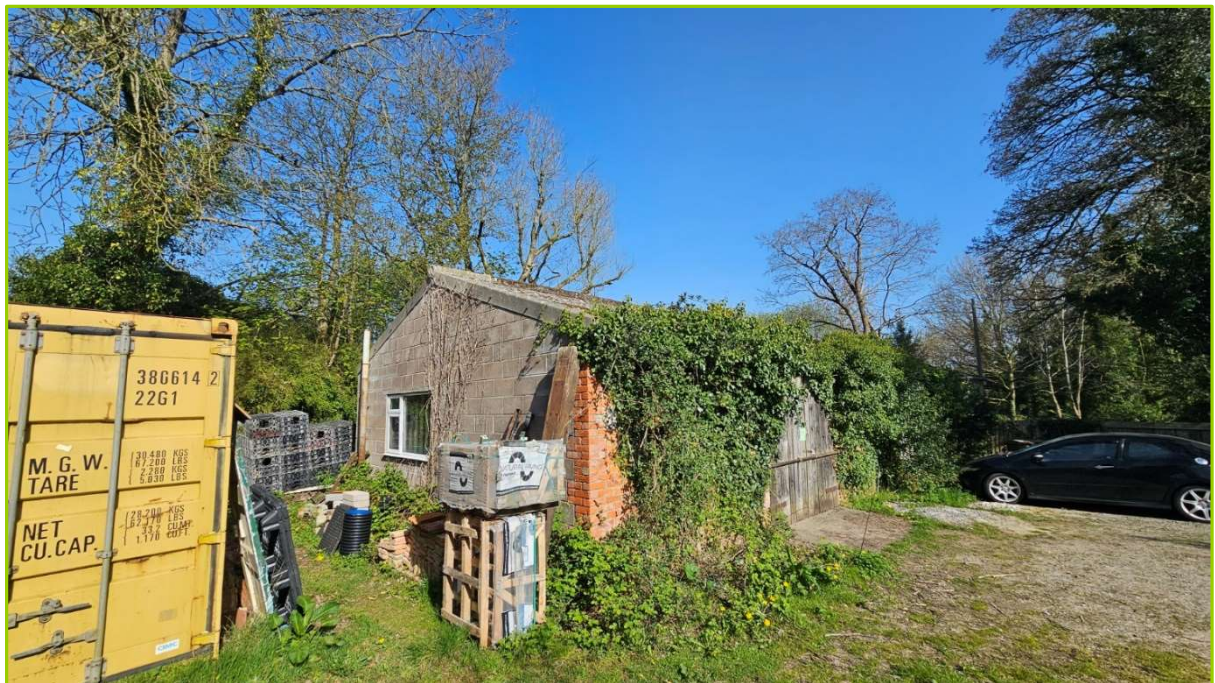
Photo 4 - View looking north showing frontage and workshop.
