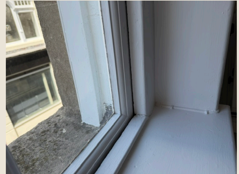
Figure 3- Internal view of the existing cable
