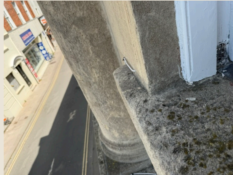
Figure 2 - External view of the existing cable
