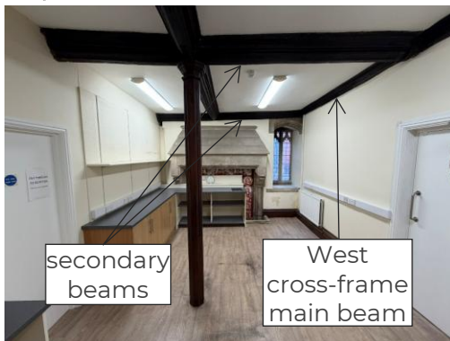
Figure 10 – Solar undercroft, looking north
