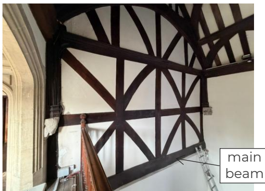
Figure 12 – cross-frame, Hall elevation
