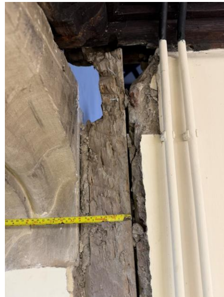
Figure 21 – general view from Solar undercroft Figure 22 – partition stud viewed within Solar undercroft
