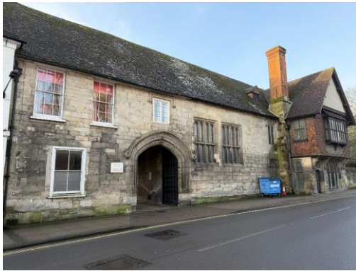
Figure 4 – north elevation, east end
