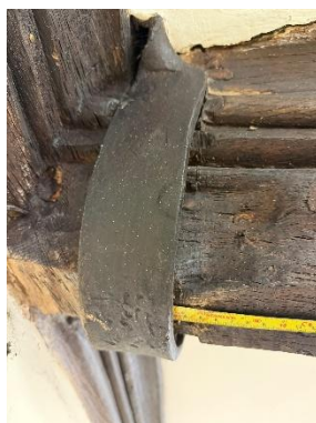
Figure 19 – central secondary beam saddle
