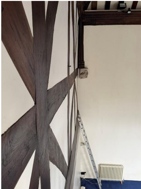
Figure 15 – north elevation, east end
