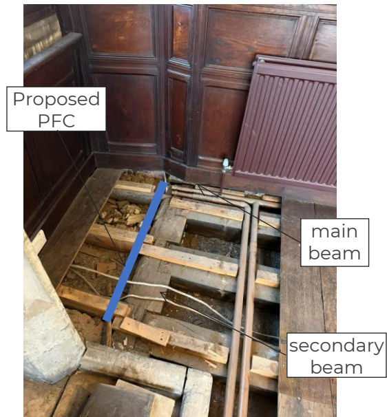
Figure 23 – beams within Solar
