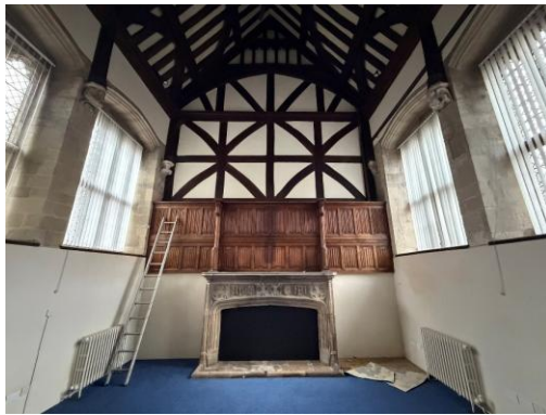
Figure 8 – east cross-frame, W elevation
