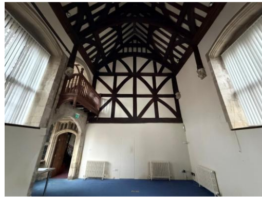
Figure 9 – west cross-frame, E elevation
