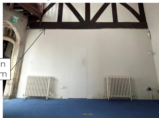
Figure 16 – partition below cross-frame, Hall elevation
