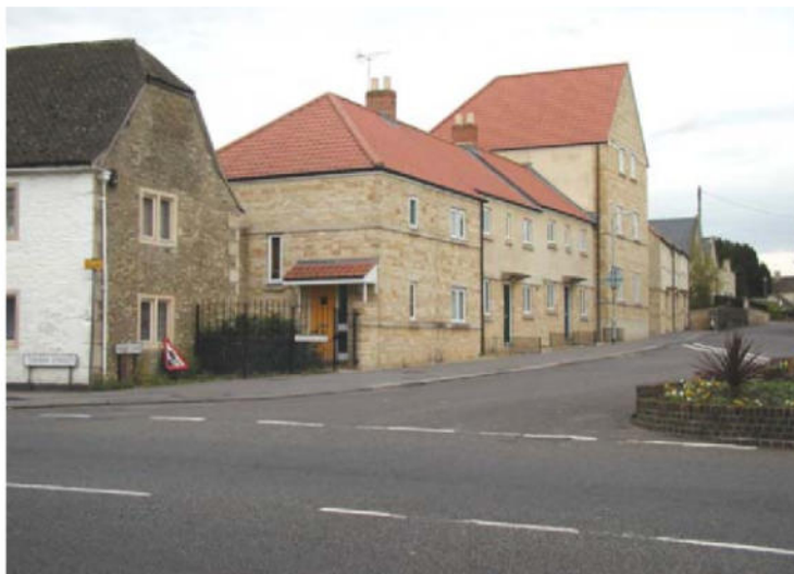
Fig 13.8: These new houses and flats do little to enhance the conservation area. The high gable is an overbearing and inappropriate feature and details such as the diminutive railing design and window units with cills that duplicate the stone cills below are examples of poor attention to detail. The roof tiles are out of place too.
