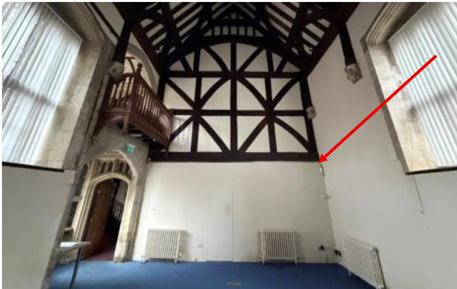
West wall of hall – position where structural is evident highlighted
