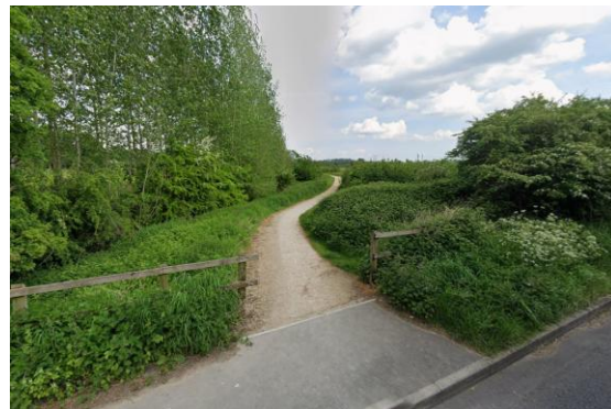
View of existing footpath to the south of the application site from West Ashton Road.
