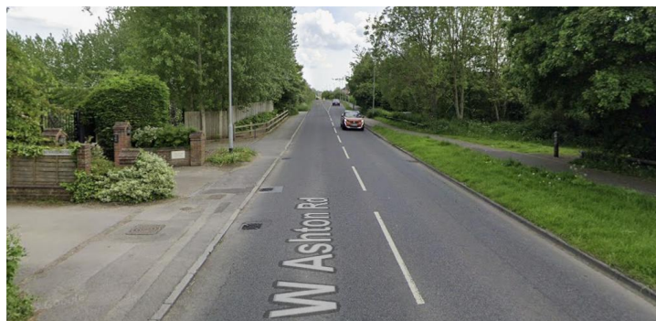
View of existing site access + southern view down West Ashton Road.
