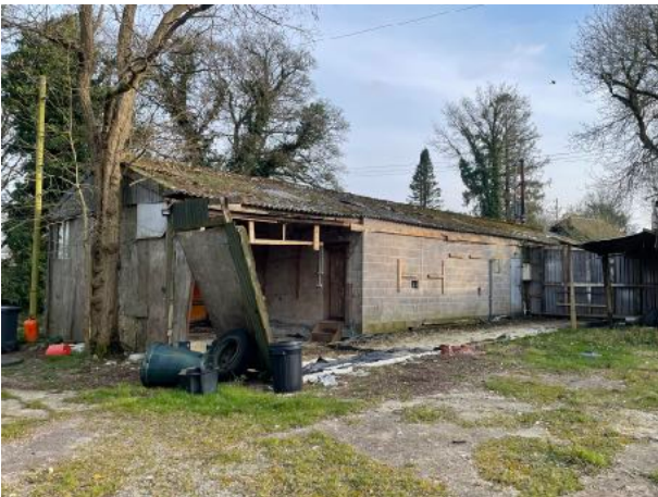
Figure 3 - Barn 1 - North and west elevations
