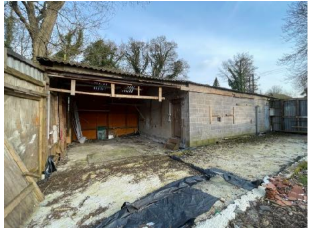
Figure 2 - Barn 1 - North elevation
