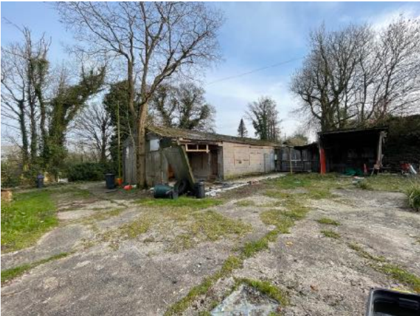
Figure 1 - Barn 1 - North and west elevations
