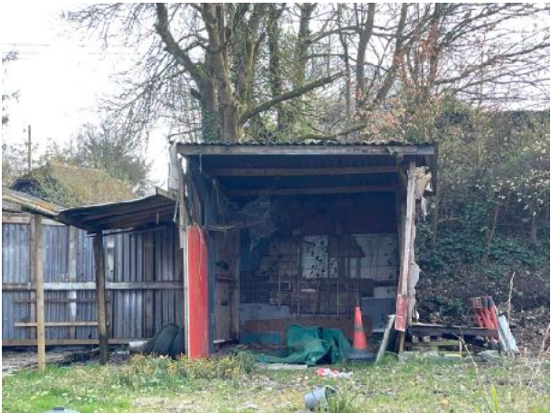
Figure 7 - Barn 2 - North elevation
