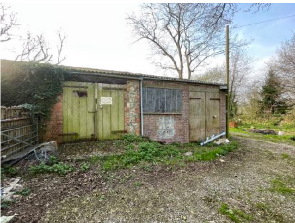
Figure 5 - Barn 1 - East elevation
