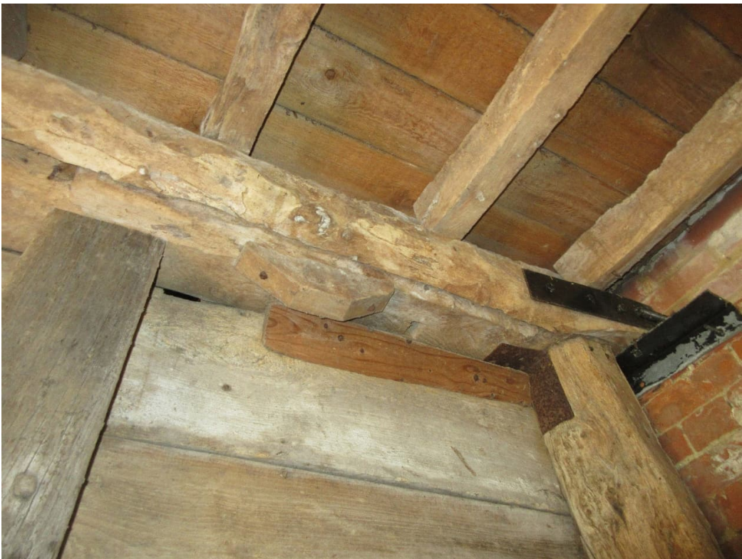
Underside detail of central truss eaves detail
