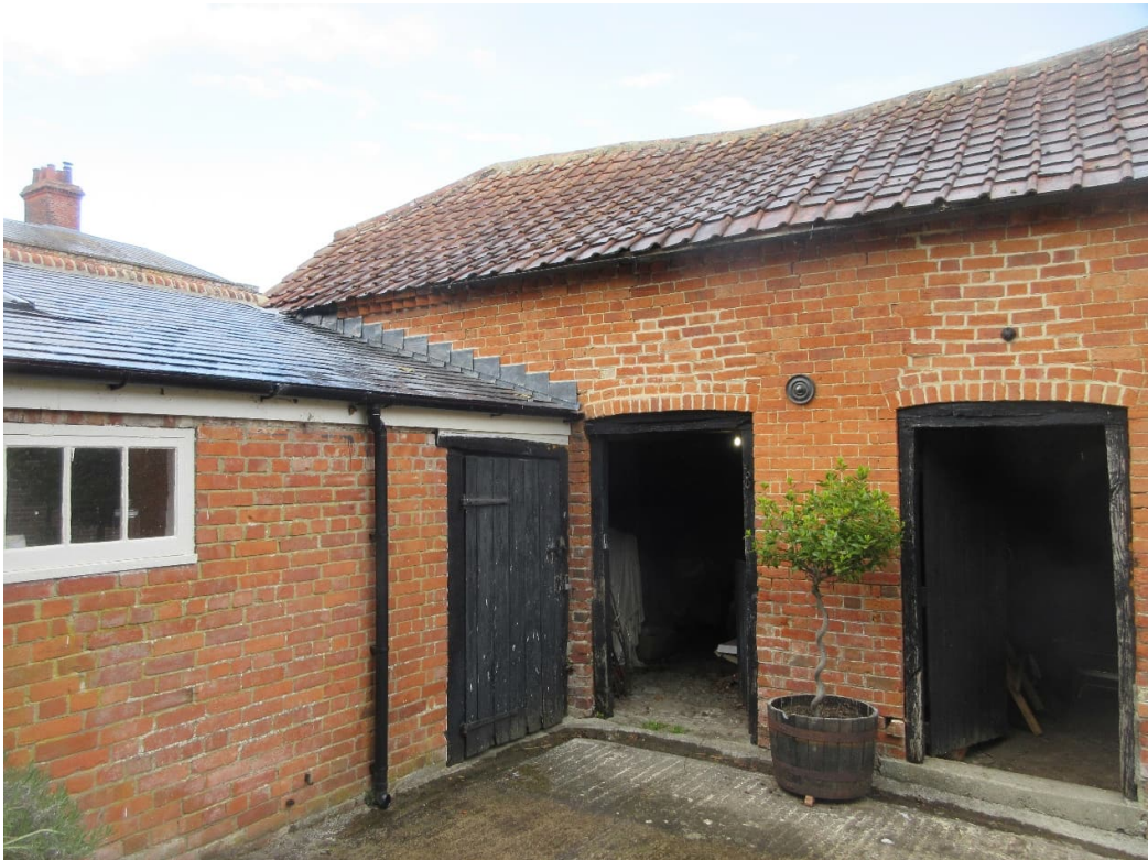
Junction of the utility wall and roof providing “buttressing” to the barn
