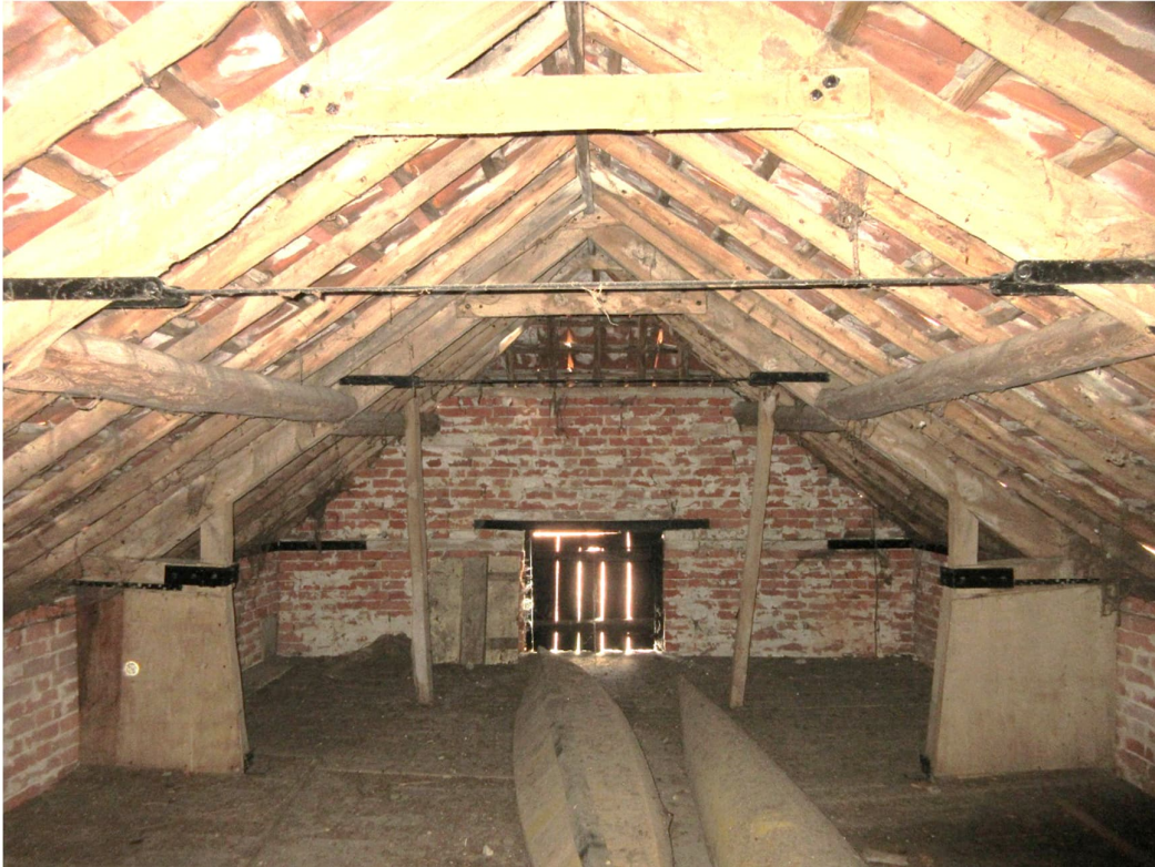
Internal view main barn first floor looking towards the east- note two hip end props and metal ties
