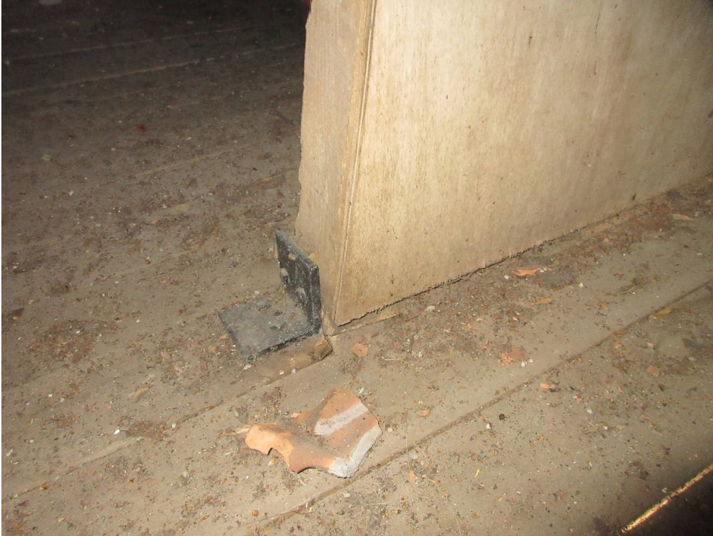
Tie down steel angle to main beams
