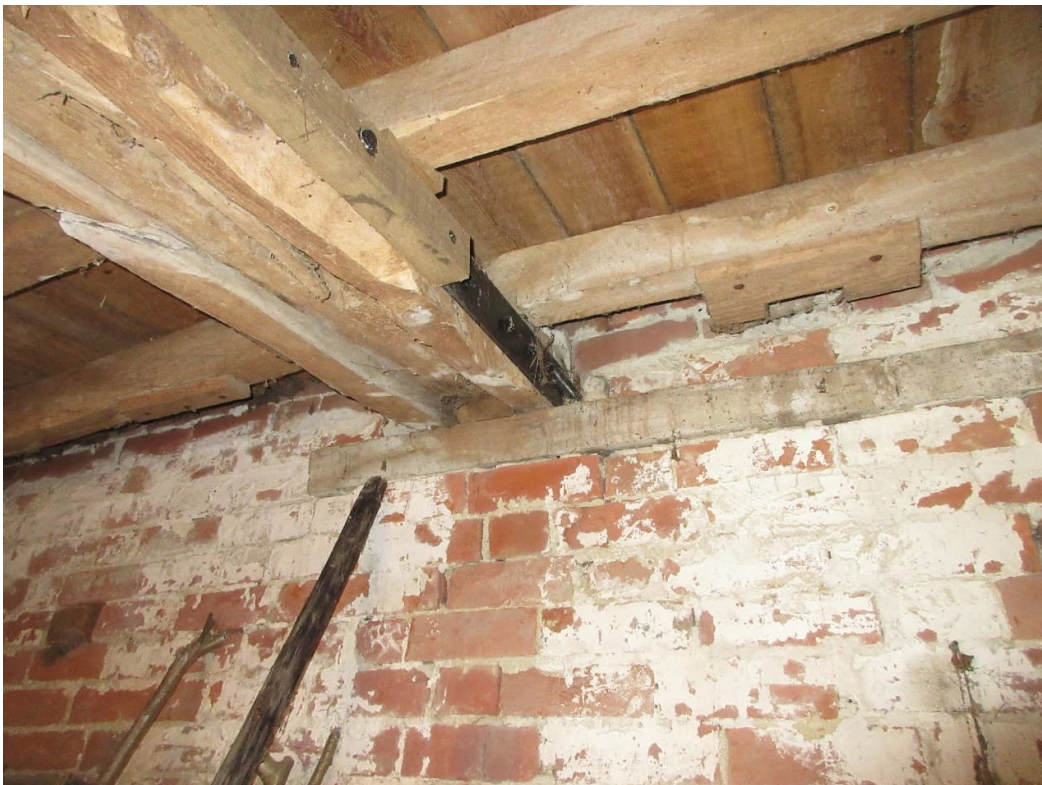
Outer side wall and beam bearing with binder
