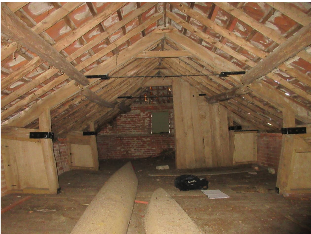
Internal view main barn first floor looking towards the west- note steel elements and ply wood diaphragms
