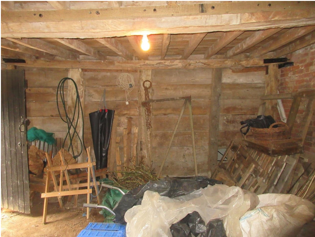
Internal ground floor view
