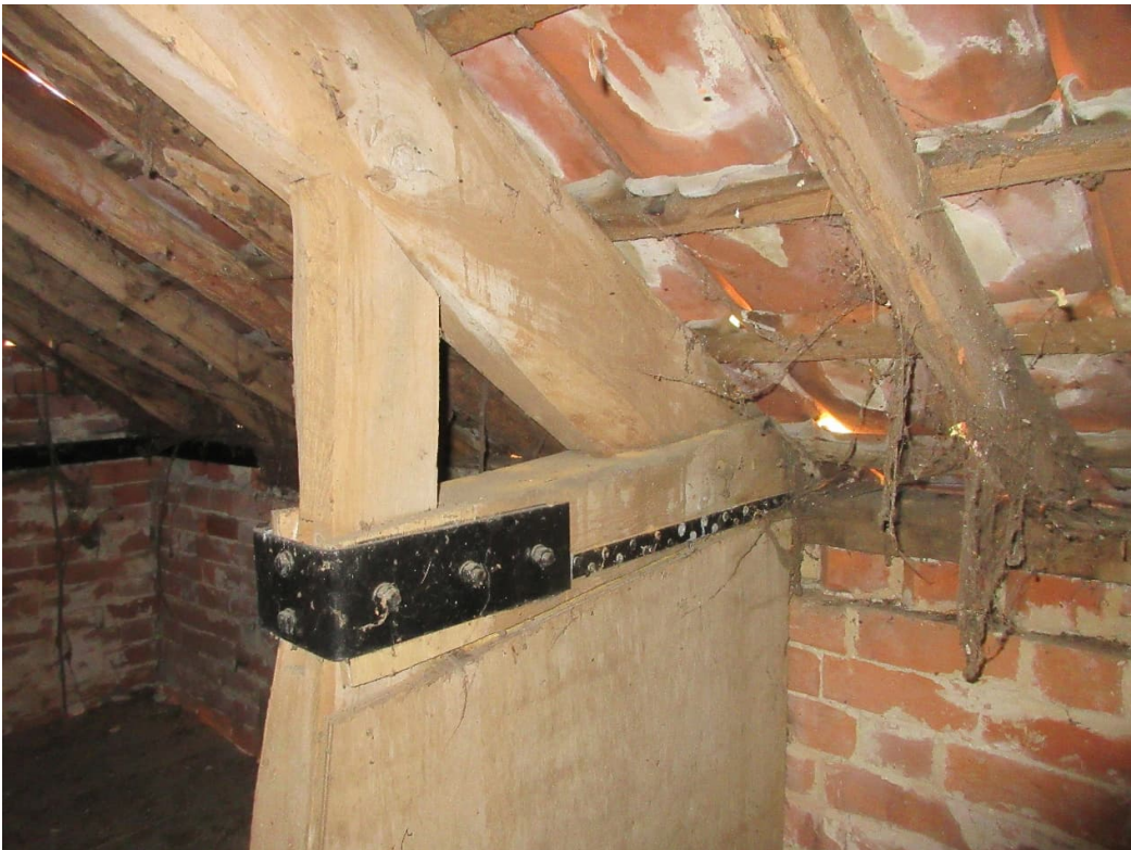
Close up opposite eaves detail
