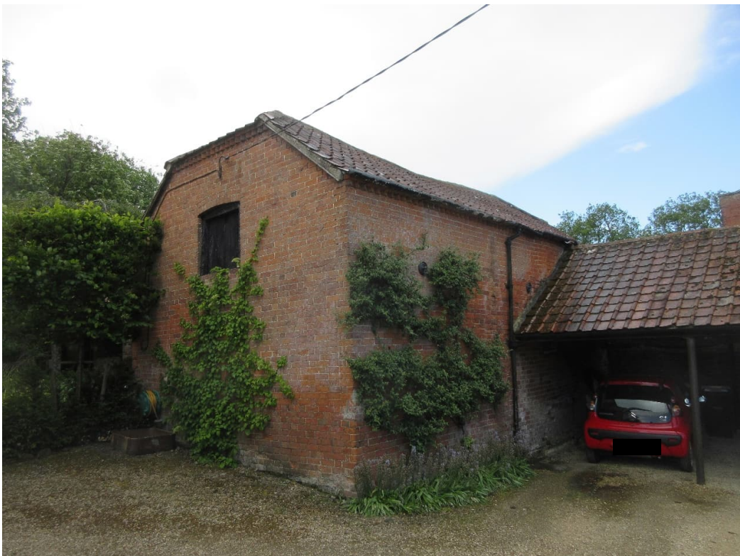
Oblique elevation east and north elevations
