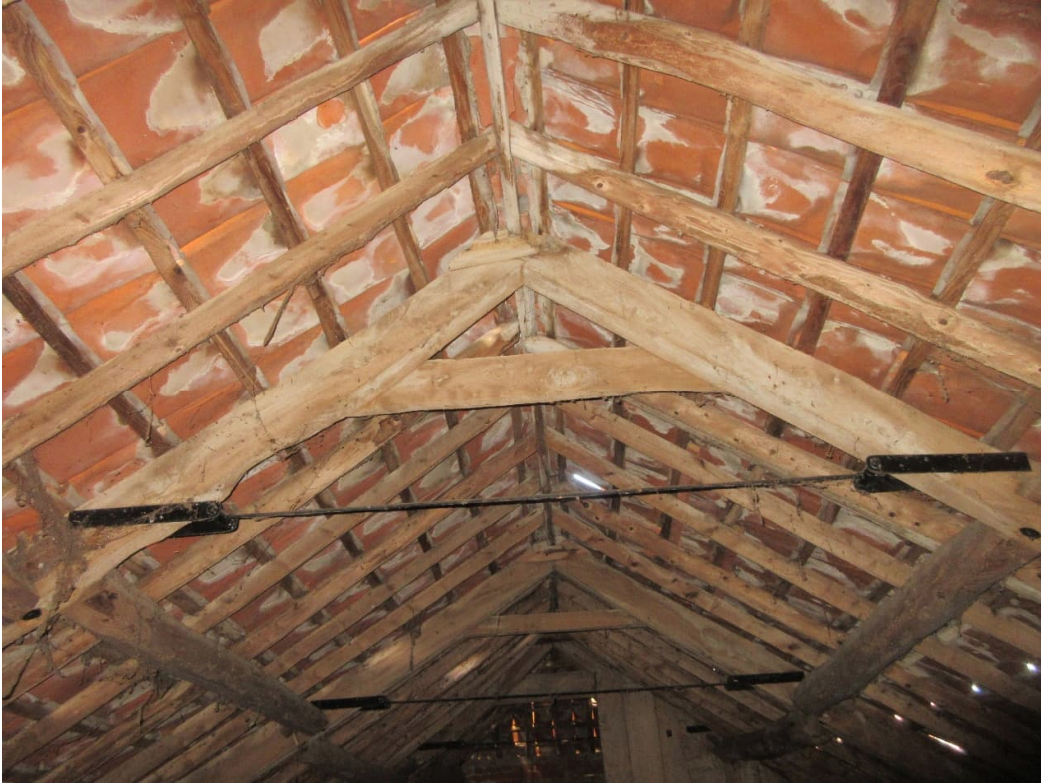
Typical truss, collar tie and lower steel tie rod
