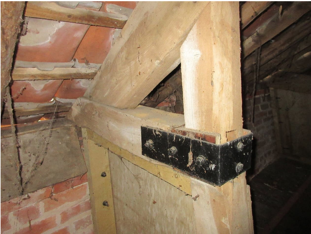
Close up eaves detail with original post and ledger and added ply wood and soft wood diaphragm and brackets
