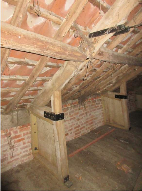
Eaves detail with original post and ledger and added ply wood and soft wood diaphragm and brackets
