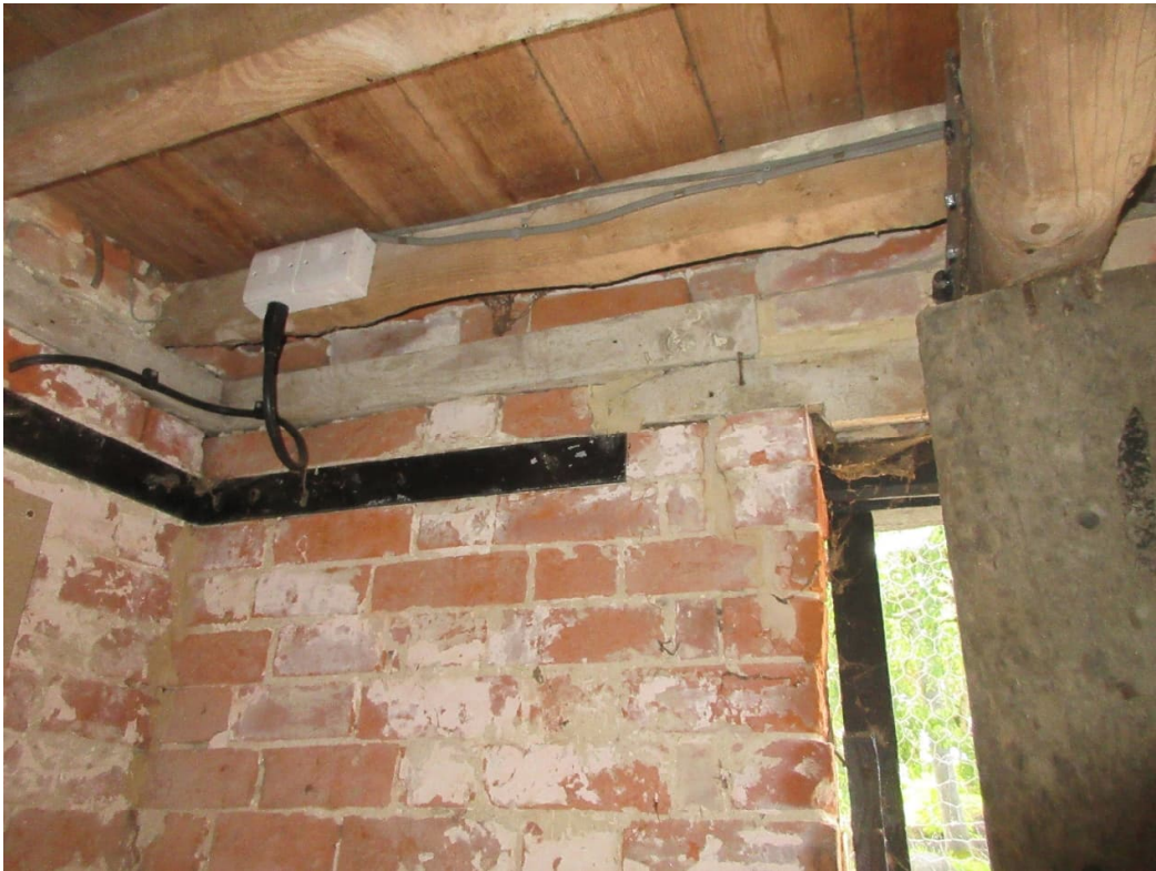
Corner steel braces
