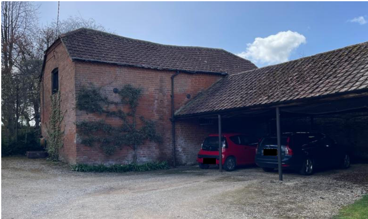
The outbuilding with its distinctive sagging ridgeline seen from High Street
