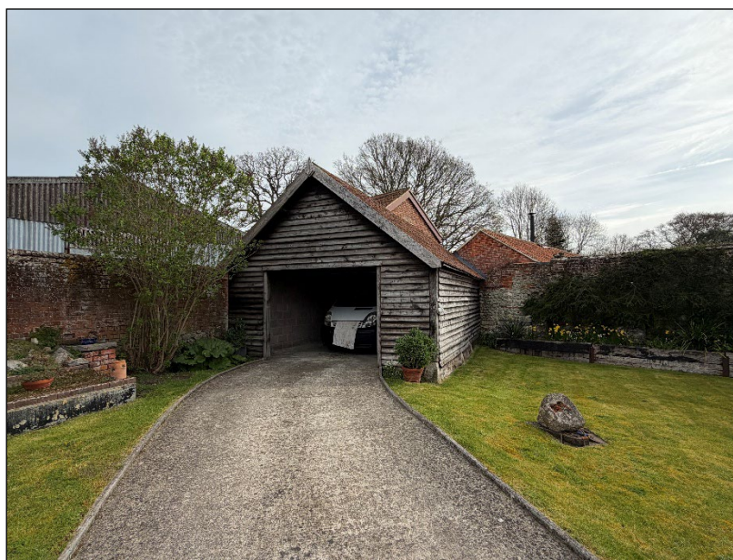
Image 17: Front elevation of garage
