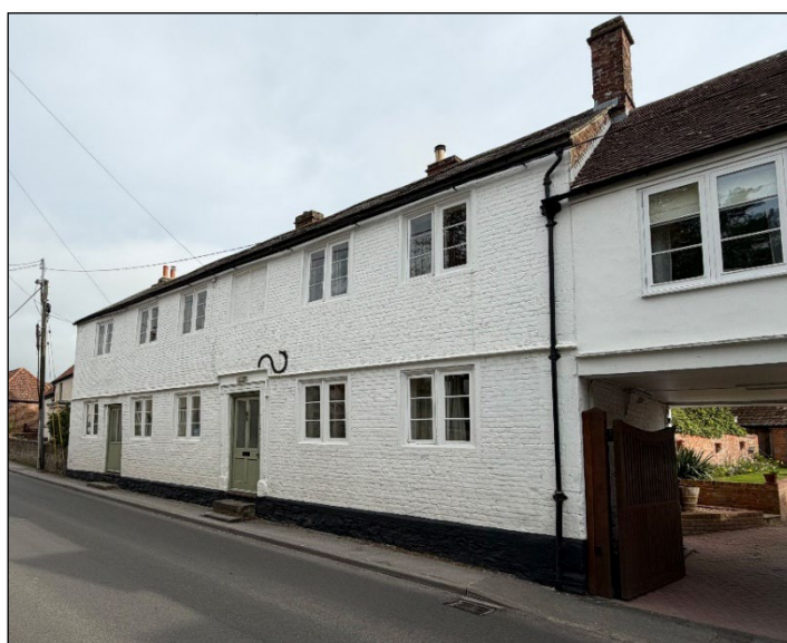
Image 22: Nos. 63 and 65 High Street, front elevation
