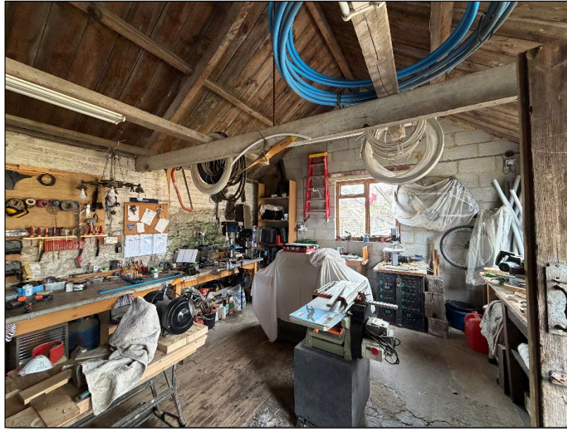
Image 16: Internal view showing replacement roof structure
