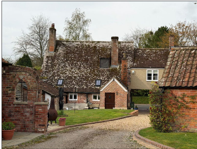
Image 19: No. 69 High Street, rear elevation
