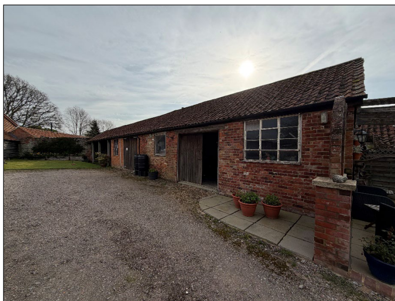
Image 14: Outbuilding viewed from southwest
