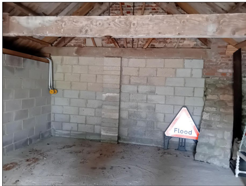
Image 13: Modern infill to rear garage wall
