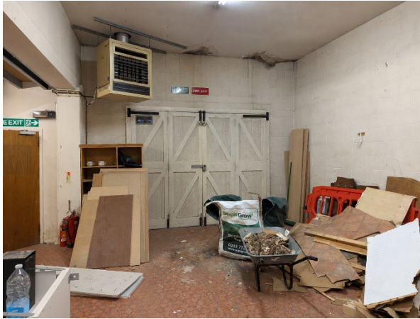
Warehouse Ground Floor
