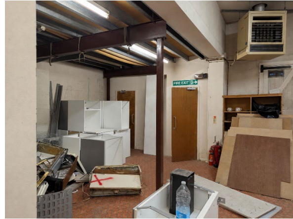
Warehouse Ground Floor
