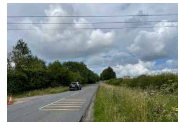
View up B4040 Common Hill / Malmesbury Road showing location of access
