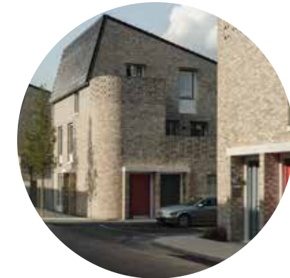
Example of a 3 storey corner turning property at prominent junction
