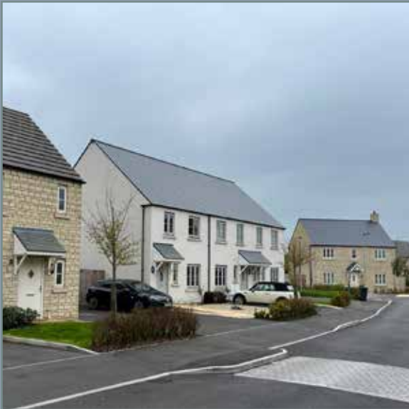
Parking and landscaping areas used to widen and create more open streets at Clover Lane, Cricklade
