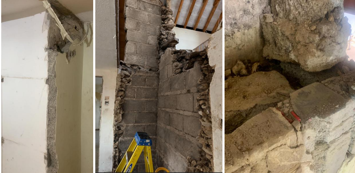
Submitted photos of internal wall during stages of opening up
