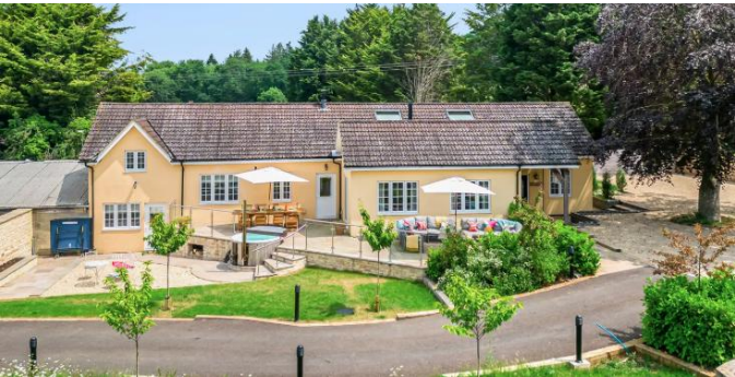
Figure 1: site photo (sykes cottages)
