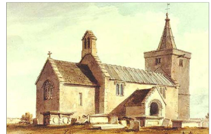
Image from www.freshford.com showing the roof over the nave as a lead roll roof and not tiles with stone.
