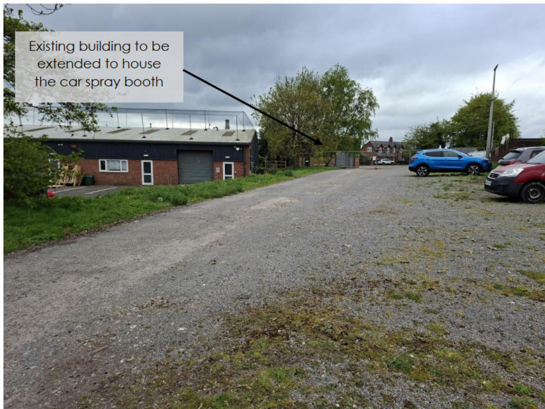
Image 3: View of building to be extended from site entrance
