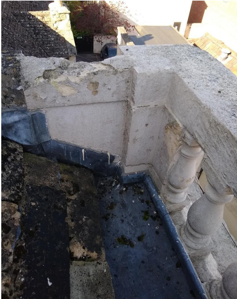
Figure 6: West end of north elevation.
