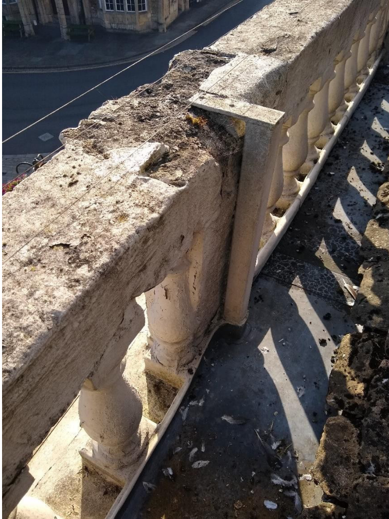
Figure 4: East elevation showing top rail and steel strengthening.
