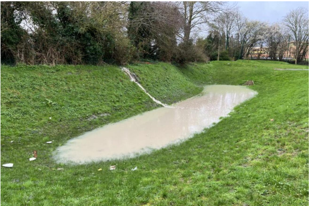
Photo 03 – Rural Runoff entering the infiltration feature as intended
