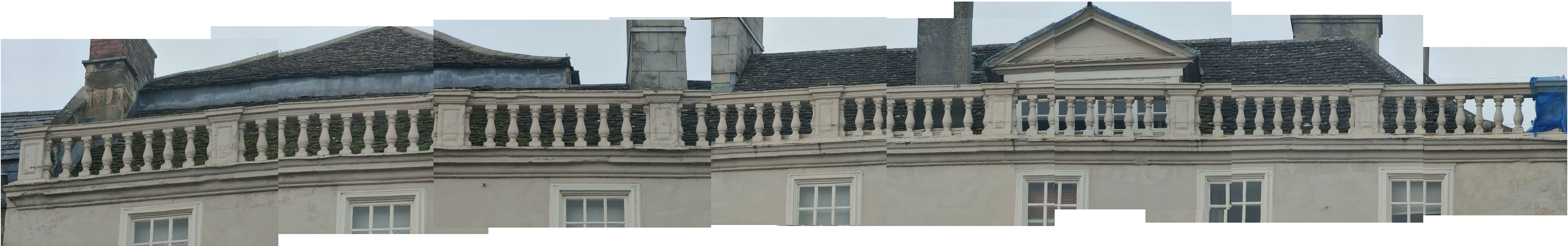
EAST ELEVATION STONE BALUSTRADED PARAPET
