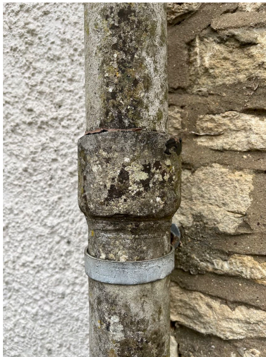
EXISTING ASBESTOS DOWNPIPE
