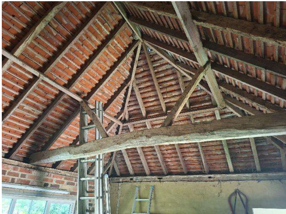
Figure 8 Interior of the western bay showing the roof truss and roof structure.
