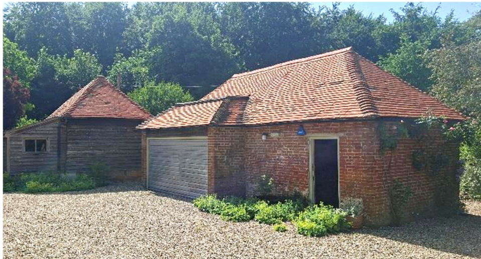
Figure 6 The garage/store building, north and west elevations, with the office building beyond.
