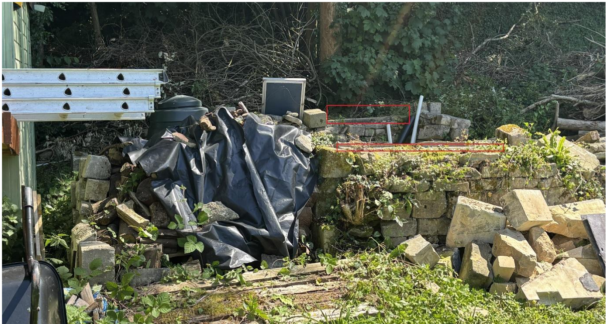
Figure 3 East Facing wall showing window ledges
