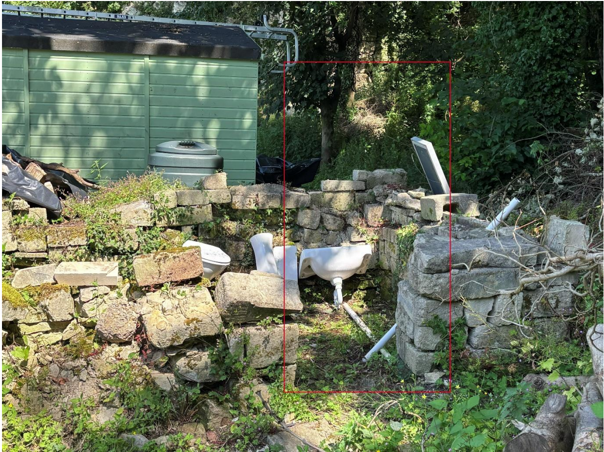
Figure 2 South East facing doorway
