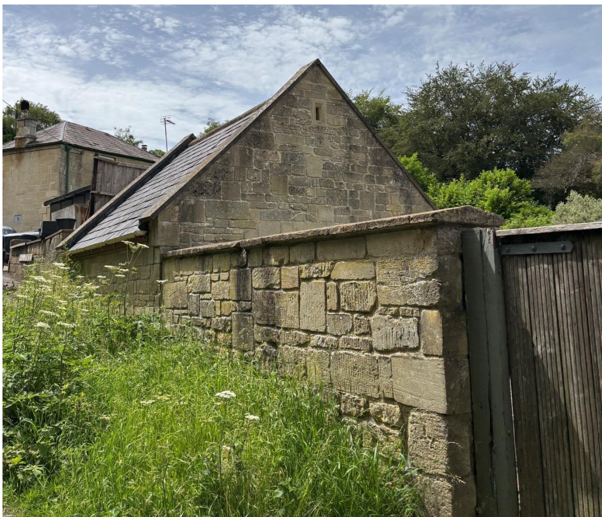
Neighbouring property with a good example of a Victorian Workshop (Barnetts Hill)
