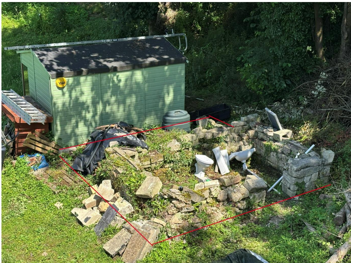
Figure 1 Outbuilding showing footprint
