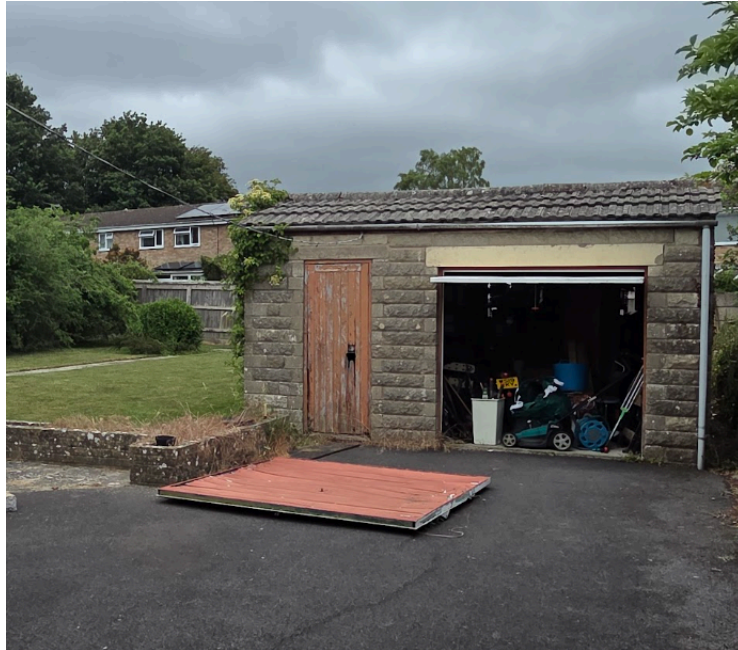
Existing detached garage
