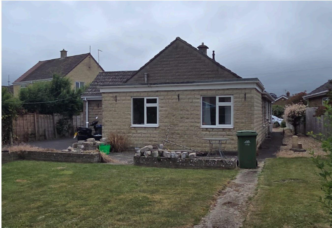
View from rear garden of flat roofed rear extension
