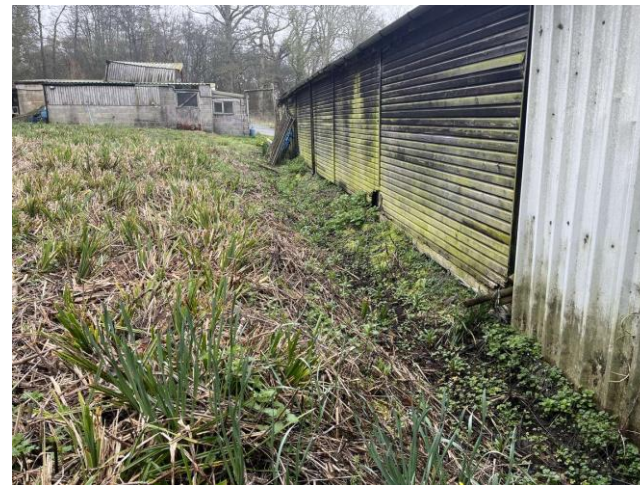
Photo 10: View of ditch behind B3.
