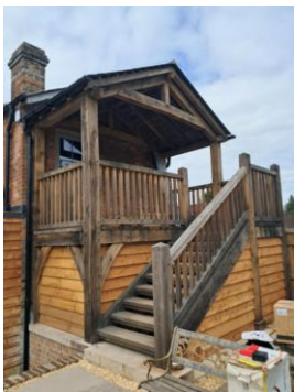
Site visit photograph showing as completed
