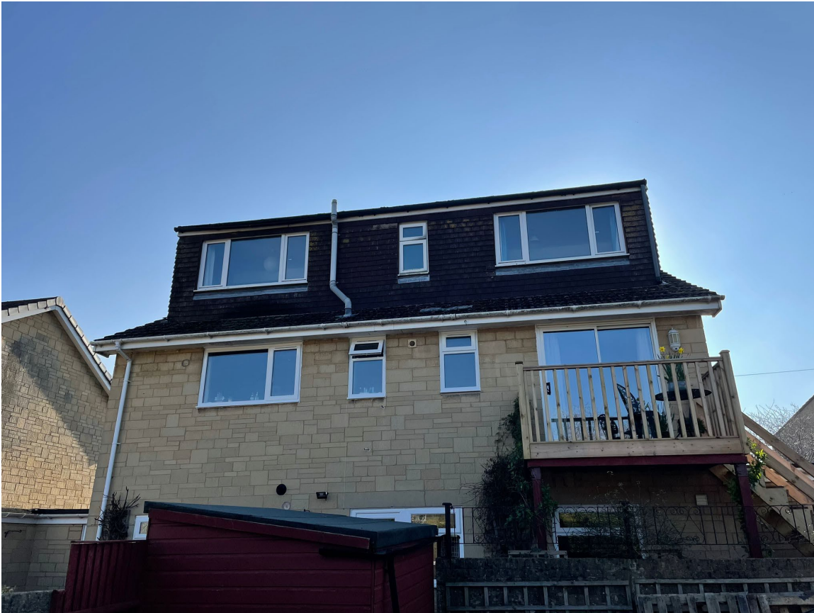
Fig. 2 – Rear elevation of property
