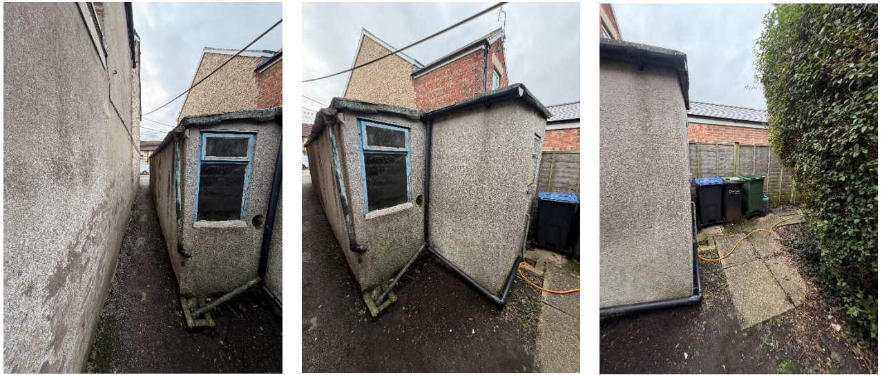
Figure 3-5: Existing rear elevations and access
