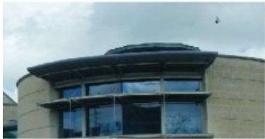
Flat roof with limestone ashlar on façade
