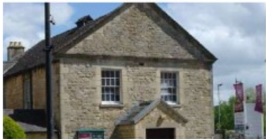
Exposed rubble stone
