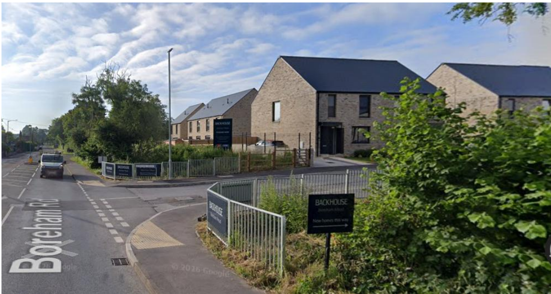
Site access to Boreham Mead further along the road
