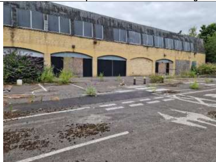
PLATE 12 – South Carpark - Site Overview – Looking West.
