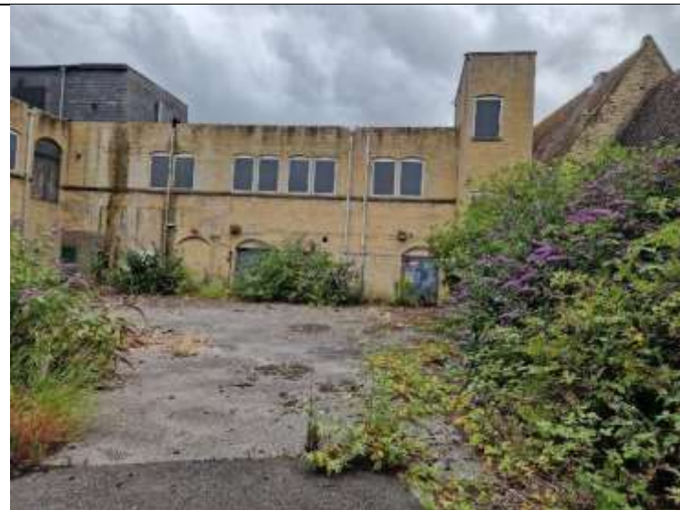
PLATE 14 – Courtyard - Site Entrance – Looking South.
