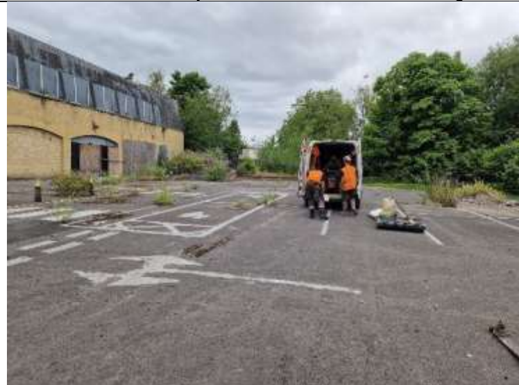
PLATE 07 – South Carpark - Site Entrance – Looking North.
