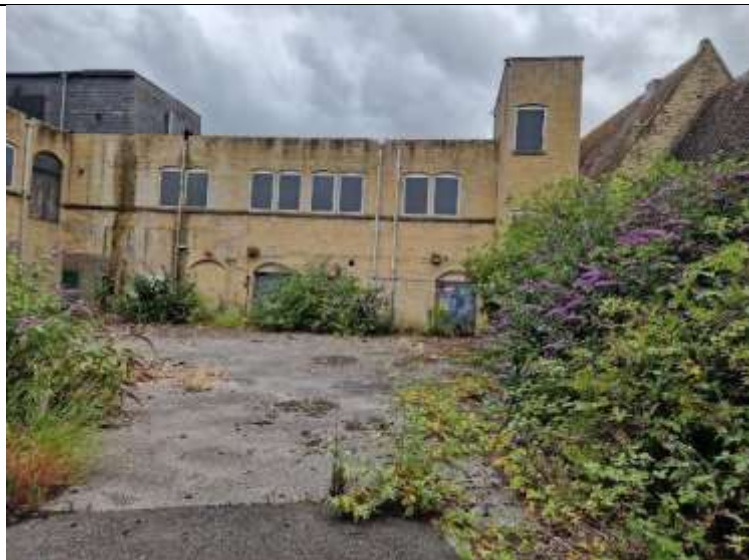
PLATE 17 – Courtyard - Site Overview – Looking South.
