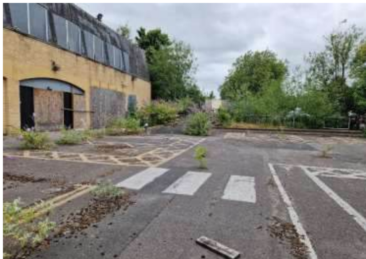
PLATE 09 – South Carpark - Site Overview – Looking North.
