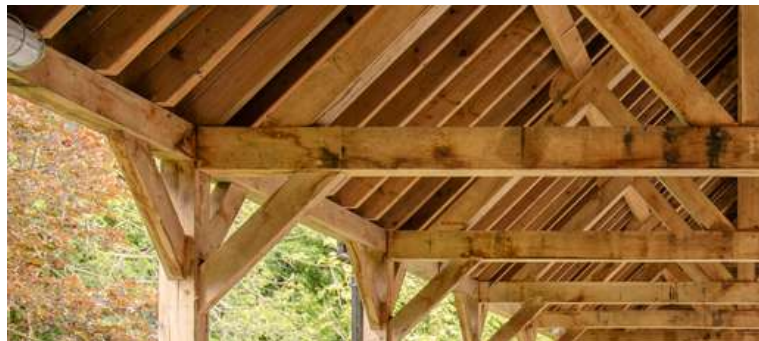
TIMBER FRAME STRUCTURE
