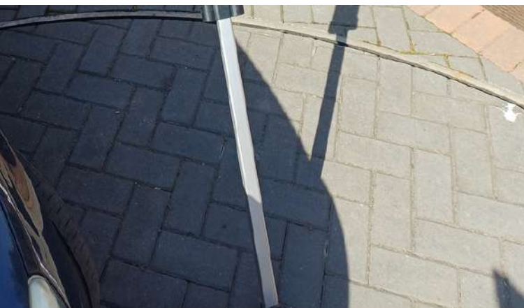
EXISTING DRIVE PAVING
