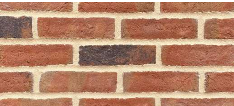
EXISTING MULTI BRICKS
