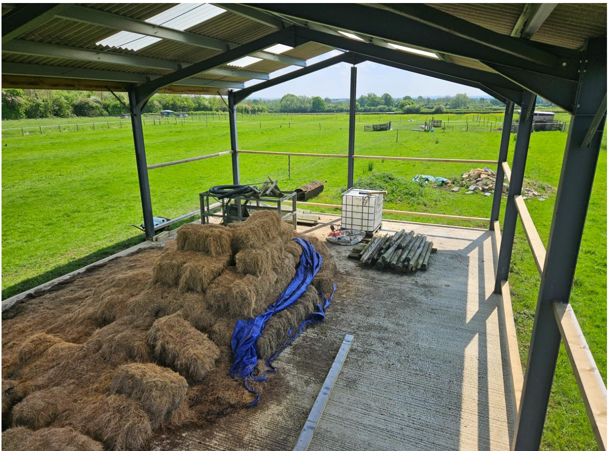
Figure 20 - The Barn with Hay (Eaten & Trampled by Sheep), Fencing materials, Chicken Runs and IBC Water Tank, May 2023
