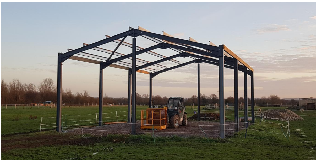
Figure 16 - Barn During Initial Construction, Sheep in Background, December 2021
