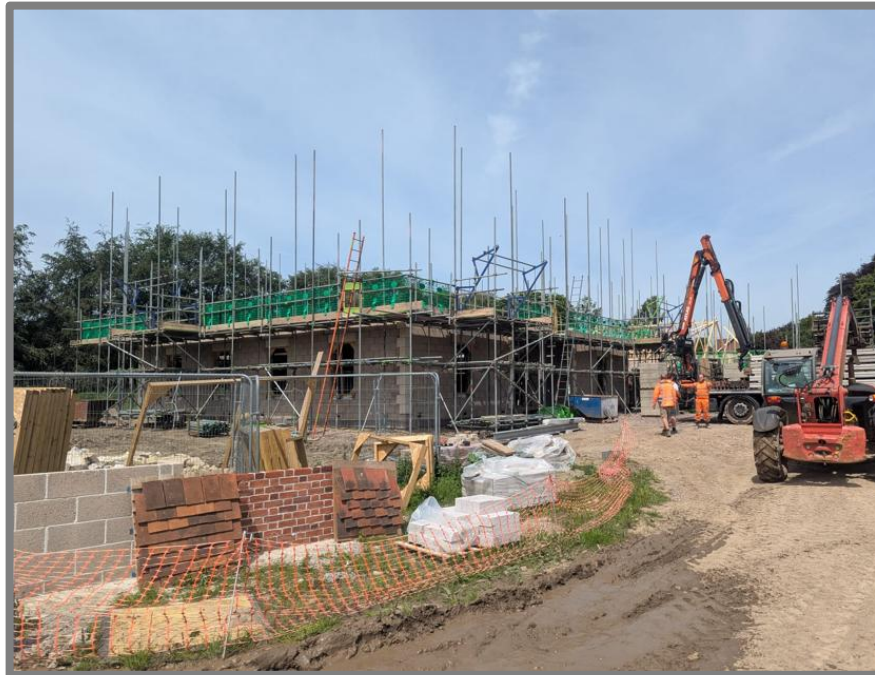
Figure 1: Photograph of dwelling under construction
