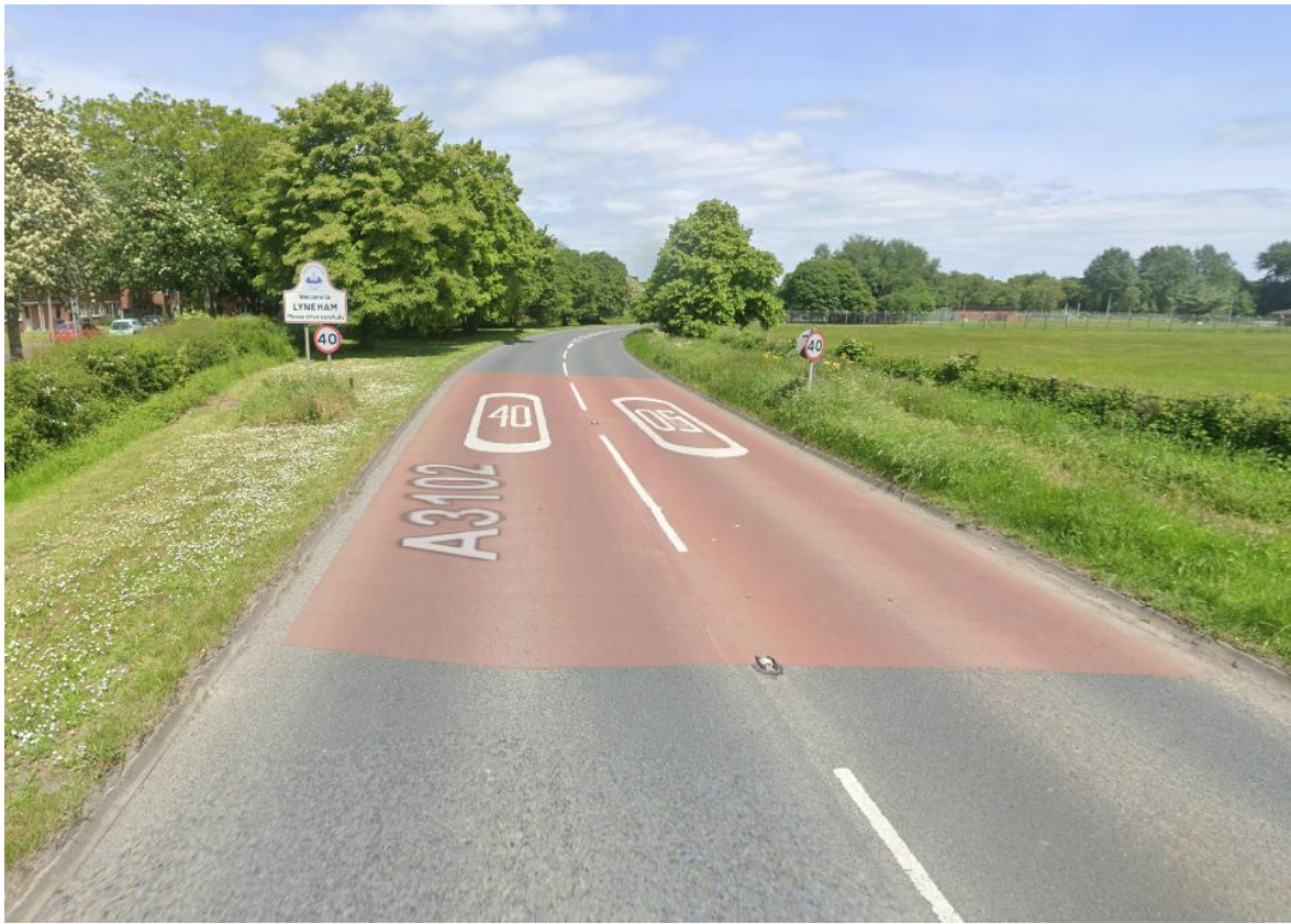
Image 2.1: Existing Gateway Feature
