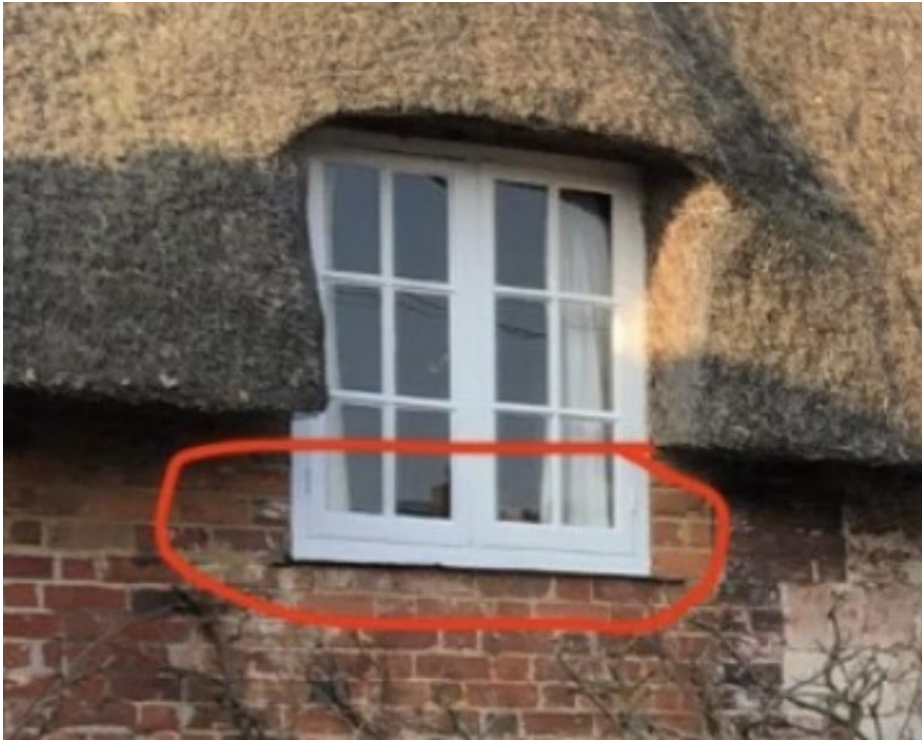
Front façade – Dormer second from left prior to replacement of single-glazed window
