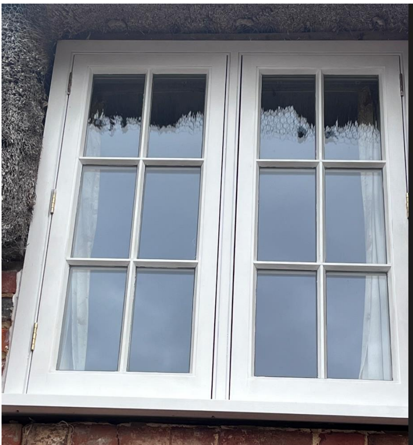
Same dormer as above with replacement double-glazed window having applied glazing bars and additional sub-cill
