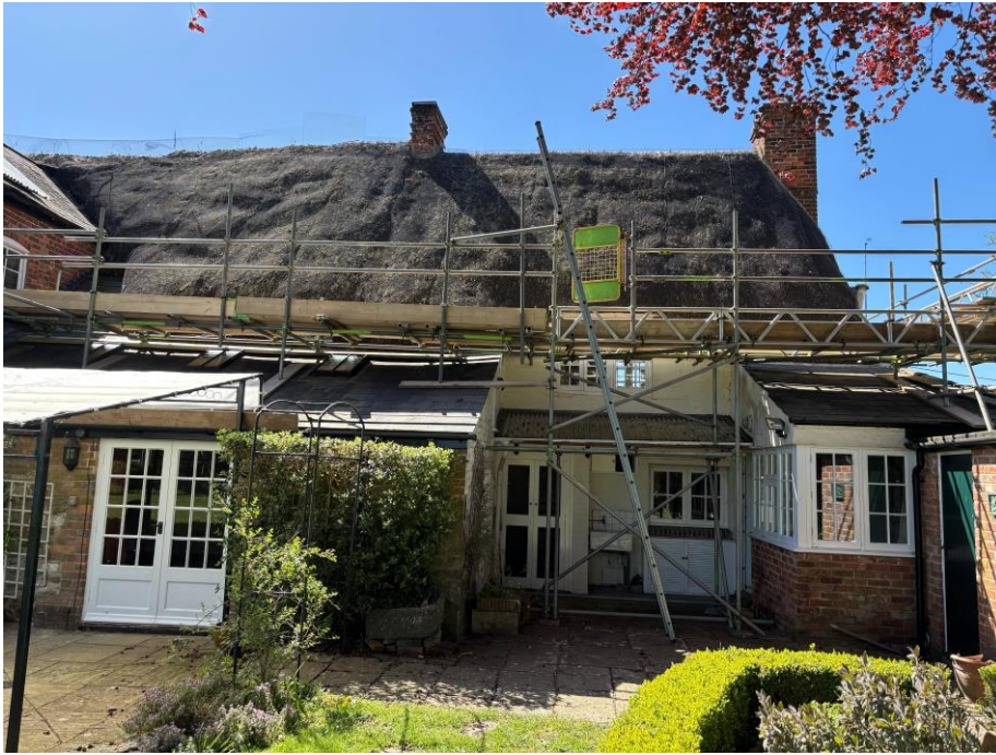
Rear elevation – c1988 utility lean-to extension on the right; older family room lean-to on the left
