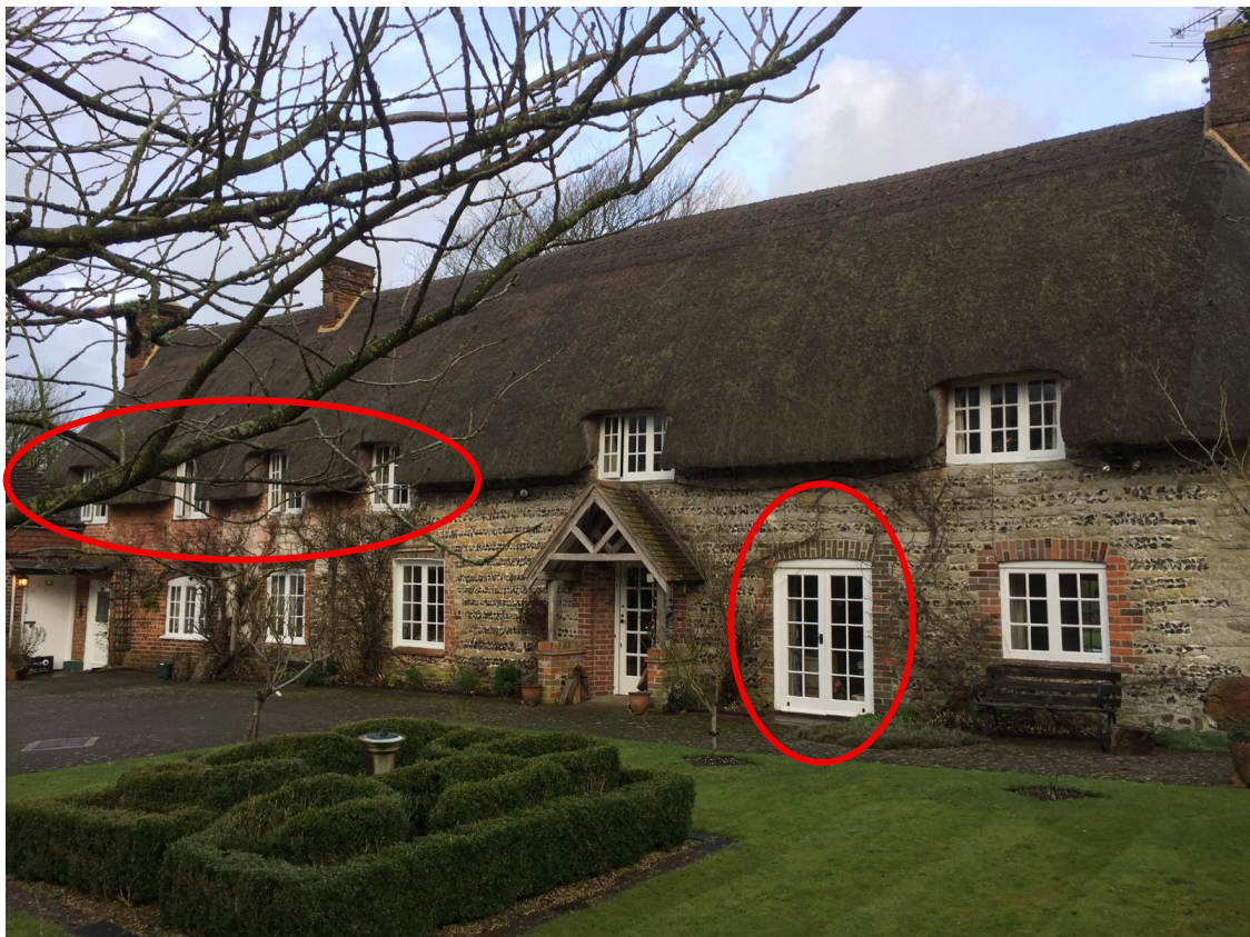
Front façade showing the four left-hand dormer windows and French doors prior to replacement
