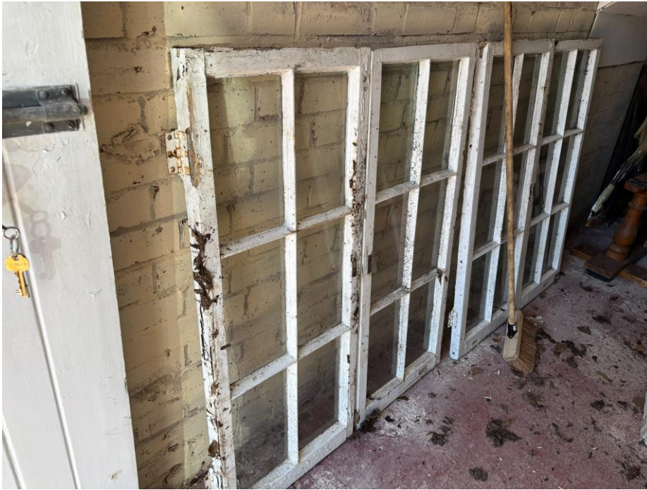
Two sets of the historic windows from the front dormers retained within the outbuilding; slender profile glazing bars (windows probably dating from the C19)
