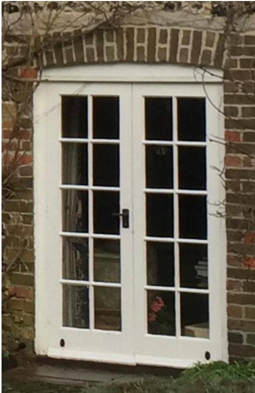
Front façade French doors prior to replacement
