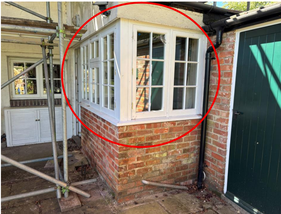
Rear elevation – Replacement double-glazed corner window in the c1988 utility extension
