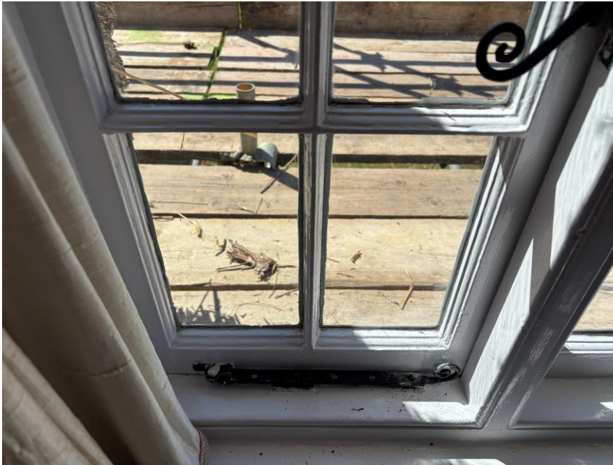
Front façade – Close up of one of the surviving casement windows from the inside showing single-glazing and fine glazing bars
