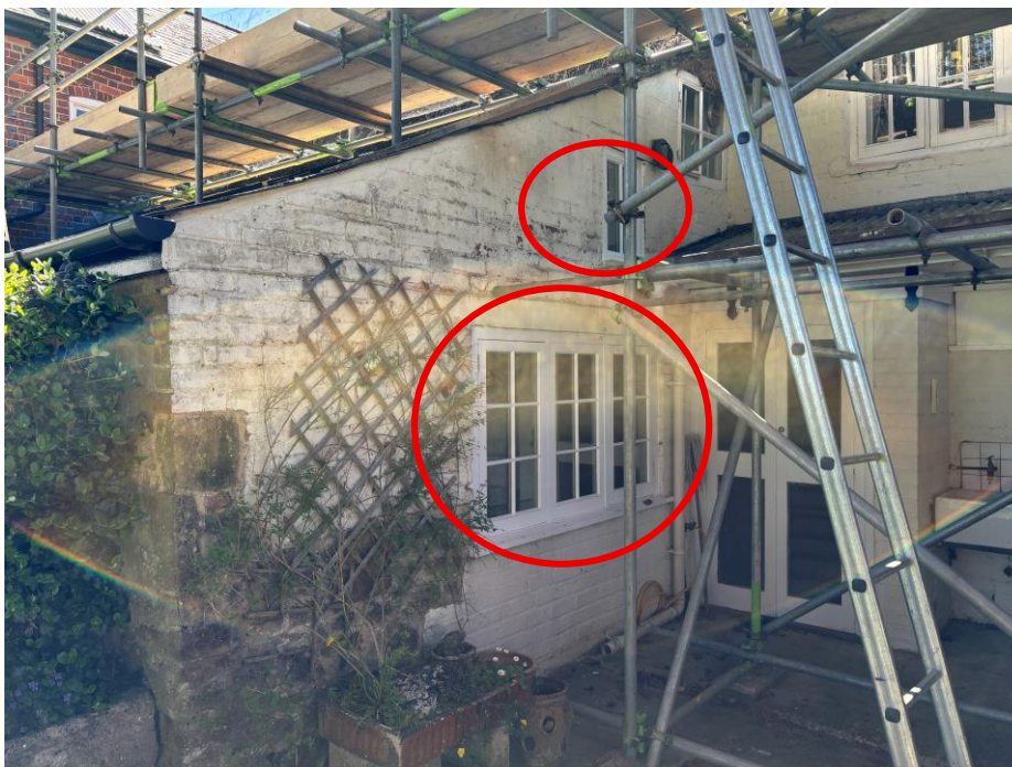
Rear elevation – Two replacement double-glazed windows in the side of the rear family room lean-to
